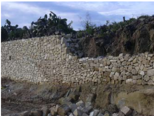
Rubble walls under re-construction.
