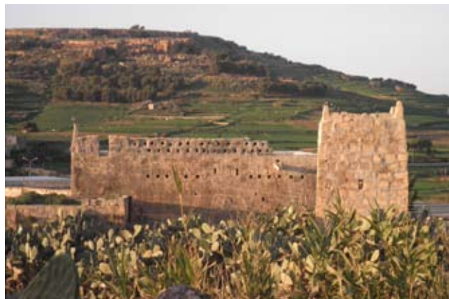
Farmhouse at Ta' Żejta Valley, Victoria showing a two-tiered screen of pigeon holes on its roof and a symmetrically laid out series of twelve corresponding nests burrowed into the wall underneath. The two smaller squarish cuts, a couple of courses further down, seem to have been intended as nests for sparrows, whereas the towering structure on the right hand side is a barumbara (dovecote).
