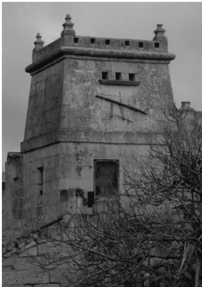
A fine barumbara at Tal-Hamrija, Xewkija. The horizontal projection serves as flying/landing platform for the nesting pigeons.
