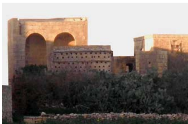
Free-standing screen wall containing five rows of around twelve pigeon holes at house in Sump Street, Victoria. The asymmetrical distribution and varying shapes of the perforations suggest the recycling of the blocks from older barumbari .
