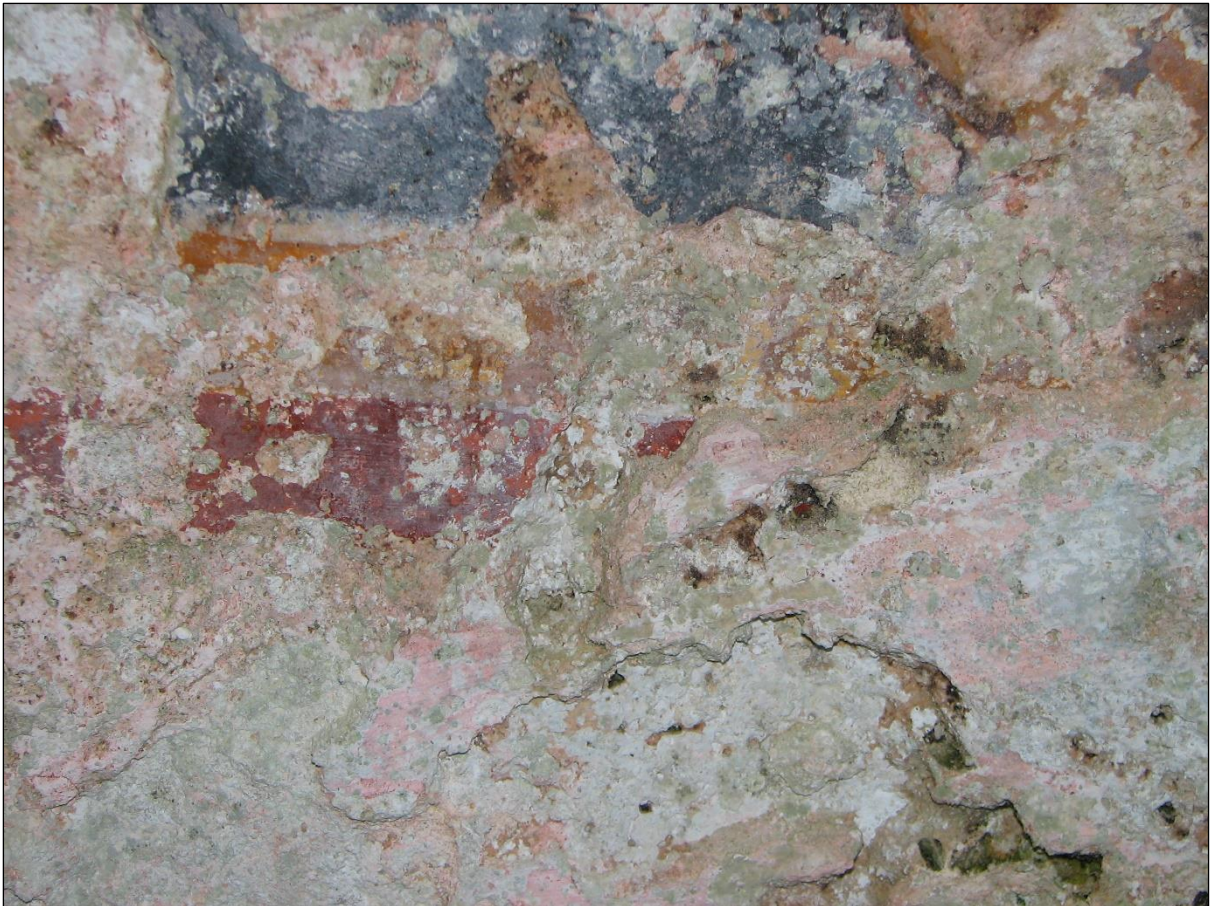
Figure 5 San Niklaw cave-church at Mellieha. Photographic detail showing two distinct coatings of painted mortar applied to the rockwall of the cave-church. Photo credit: K. Buhagiar.
