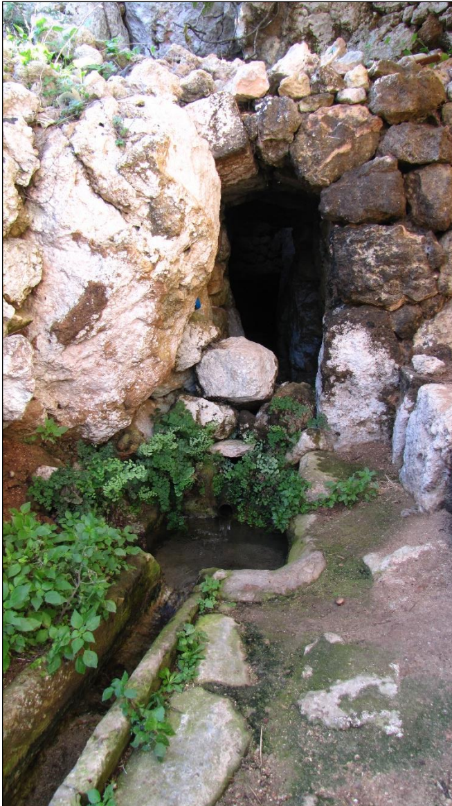
Figure 3 Gnien San Niklaw, Mellieħa. The dry-stone built entrance section to the water gallery providing this agricultural estate with a perennial water supply. Water is conveyed to different areas of the valley by means of masonry canals. Photo credit: K. Buhagiar.
