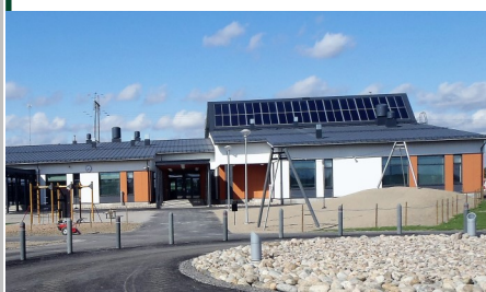
Solar collectors integrated into the roof of a school in Lapua. FP7, Concerto Photo by Pauli Kortesoja
