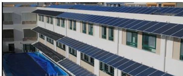
Unglazed pool solar thermal system & PV overhangs (Malta)
