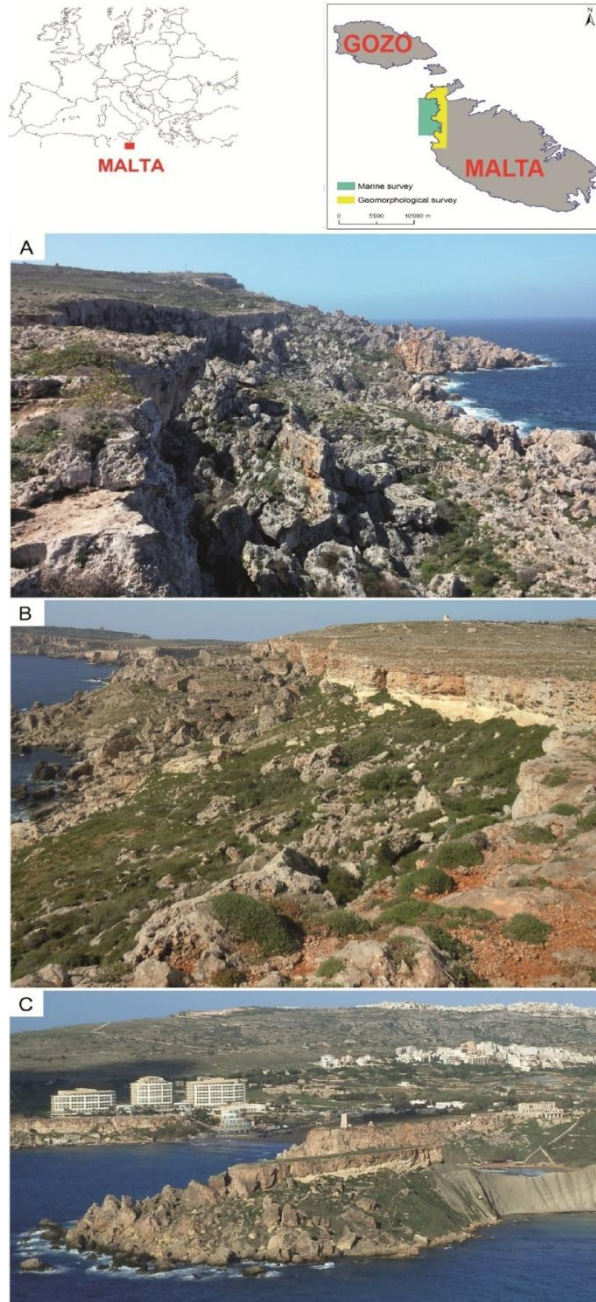
Figure 1. Geographical setting of the investigated area and examples of block slides: A) north-western area of Marfa Ridge; B) stretch of coast between Rdu id-Delli and Ras Il-Wahx; C) Il-Qarraba peninsula.
