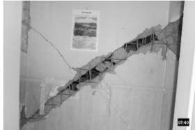
Longitudinal shear wall crack
