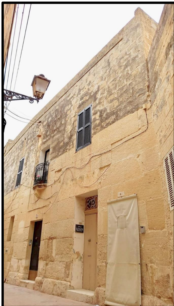
Figure 31. Photo showing the ashlar masonry wall in Triq Karmnu (Wikimedia).
