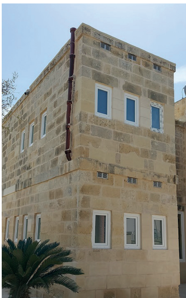
Part of the back of the campus after restoration.
