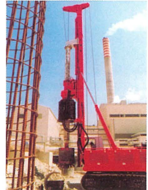
Piling works for Enemalta, gas turbine foundations
