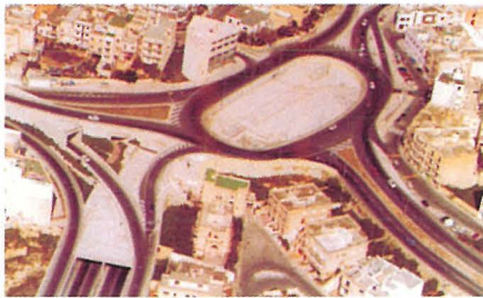
Msida multi-level intersection
