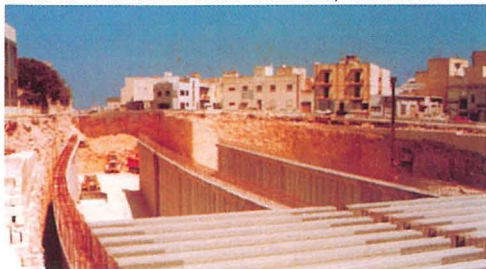
Msida multi-level intersection
