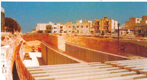
Msida multi-level intersection
