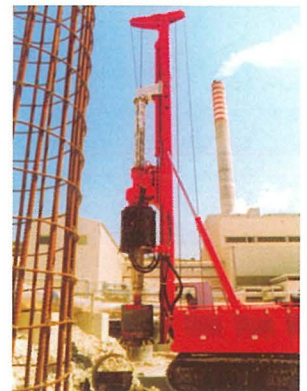
Piling works for Enemalta, gas turbine foundations
