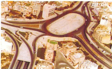
Msida multi-level intersection
