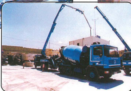
RMC and Concrete Pump
