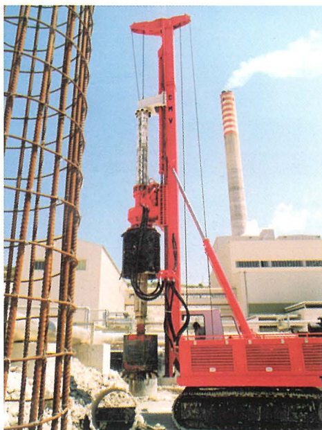
Piling works for Enemalta, gas turbine foundations
