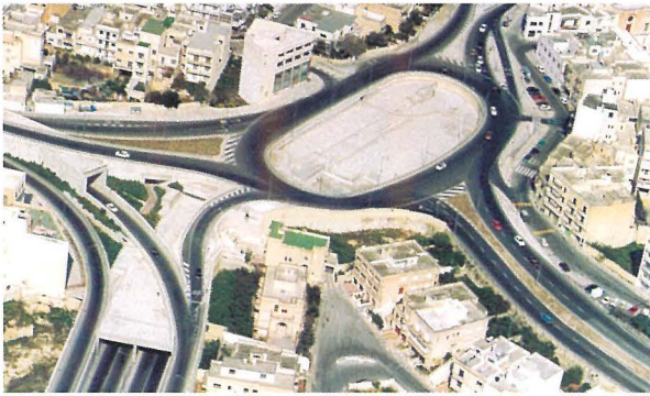
Msida multi-level intersection
