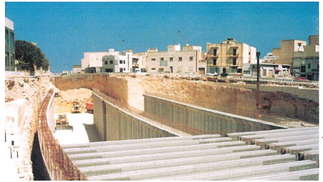
Msida multi-level intersection
