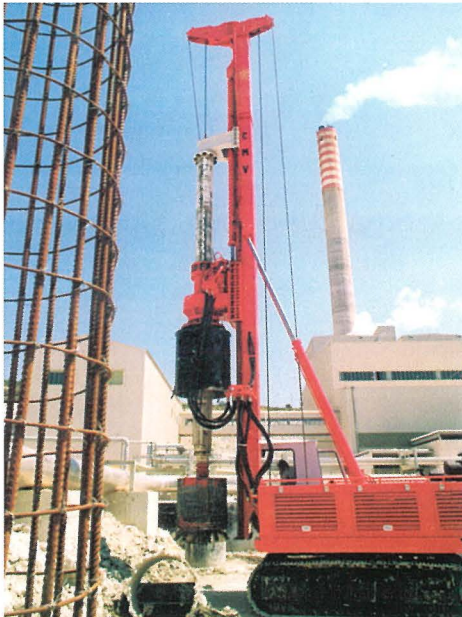
Piling works for Enemalta, gas turbine foundations
