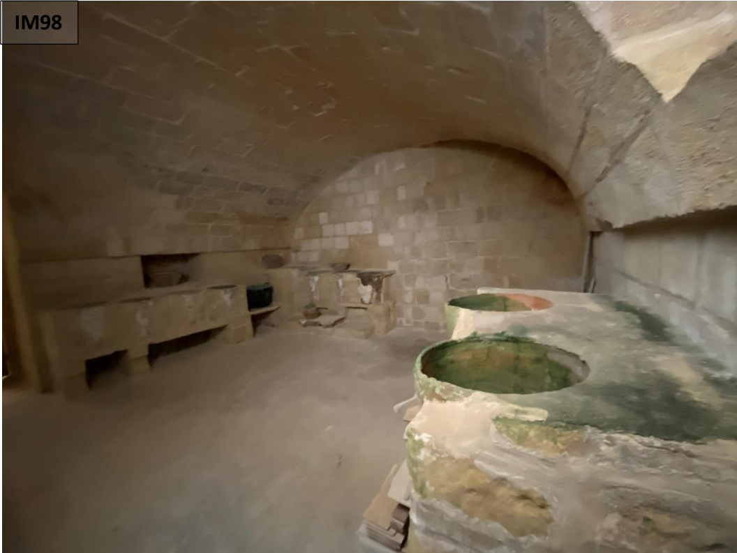
Areas with troughs and terracotta moulded basins reserved for storage or manual labour
