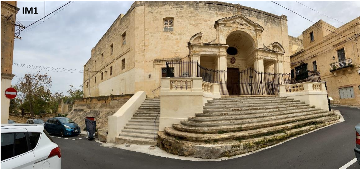
Façade: Entrance to parlour (left). Portico to Church (right)
