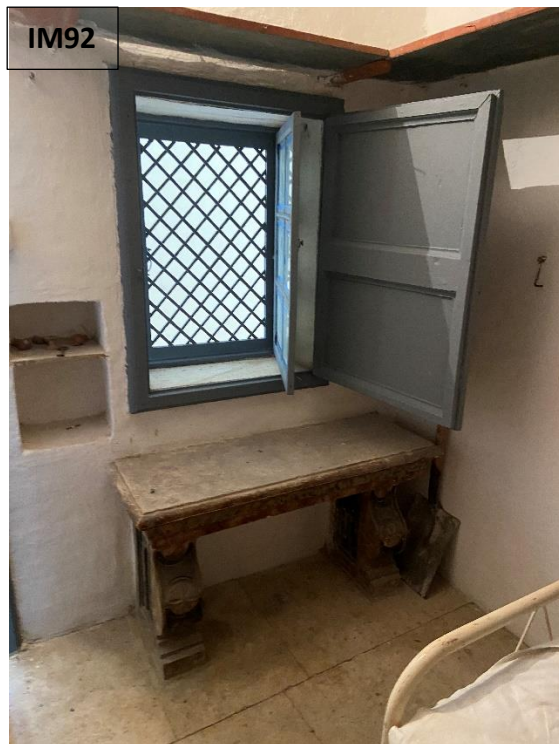
Detail - Window onto corridor in cell
