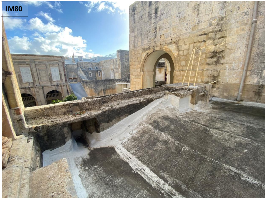
Area intended for washing laundry on the roof (Caruana Dingli, VC, 2022)
