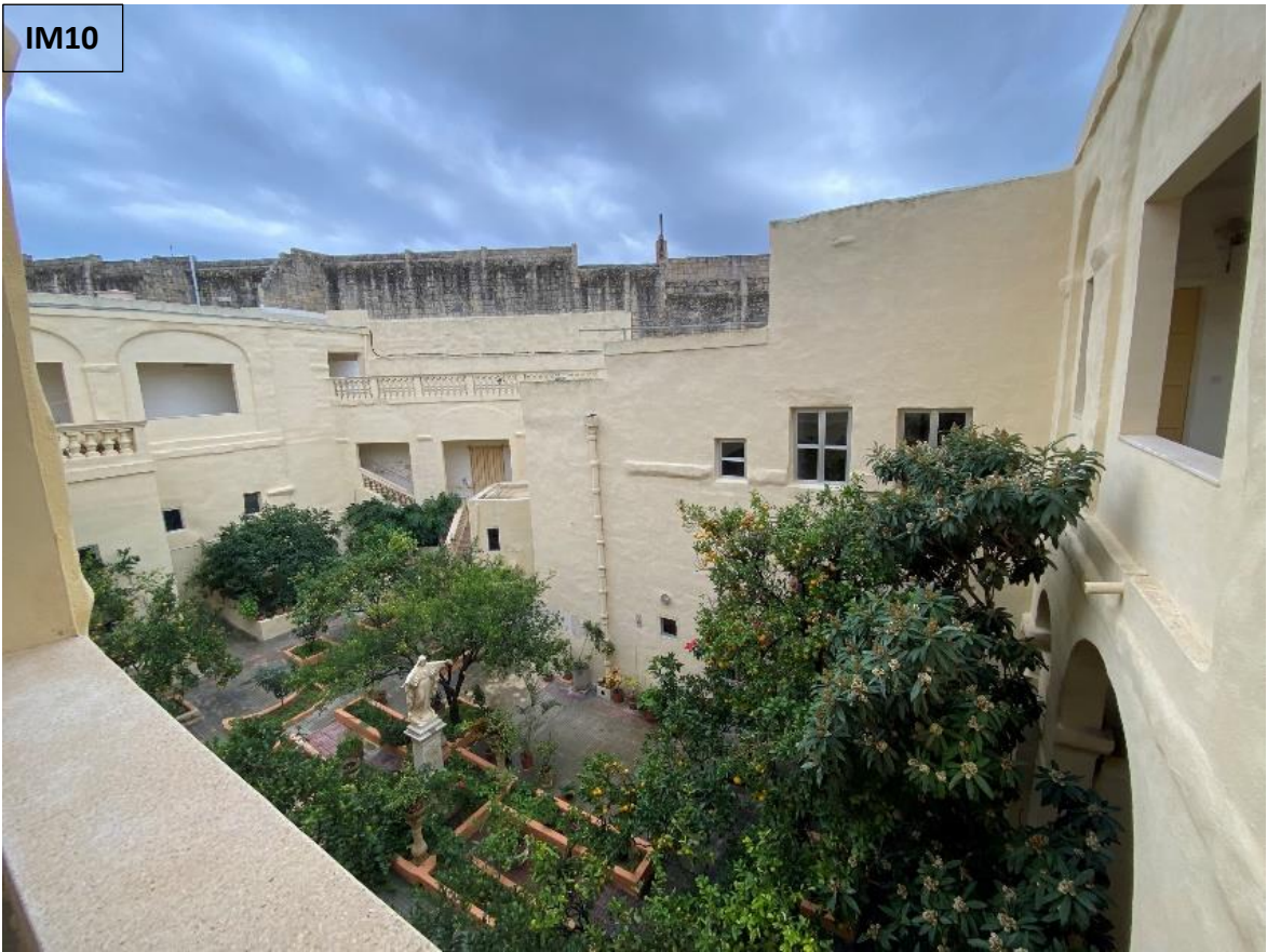
View of enclosed garden from second floor loggia
