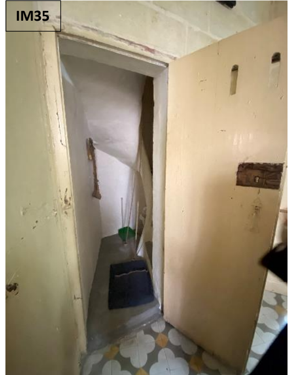
Spiral staircase to belfry. Ropes presumably used for mortifications seen hanging on the walls.
