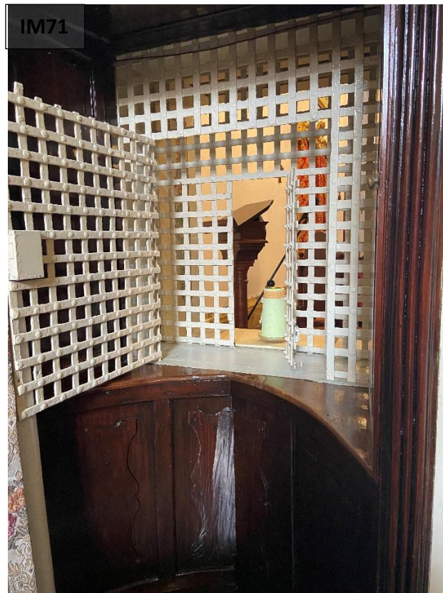
Communion window with double grille still in place
