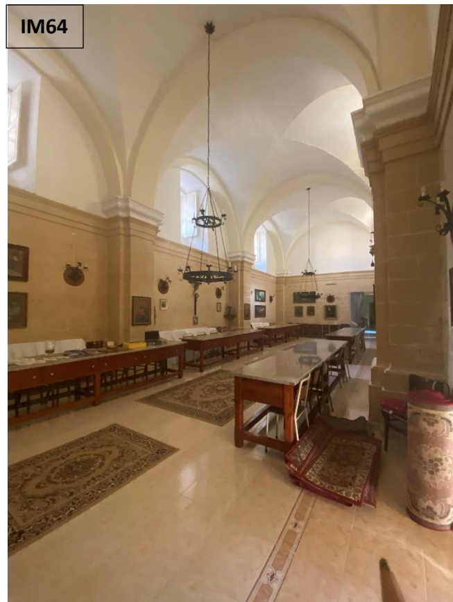
Refectory with quadripartite vaulted ceiling attribute to architect Lorenzo Gafa (Buhagiar & Fiorini, 1996)
