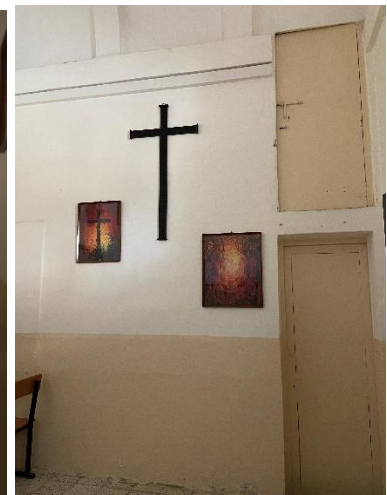
Figure 23. Access to church at ground floor level and to musician's balcony above.
