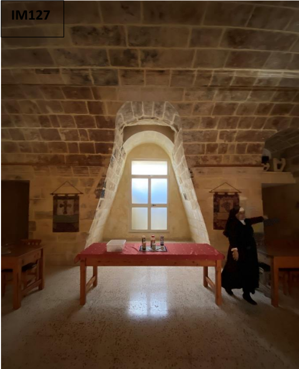
Old chimney flue of former kitchen
