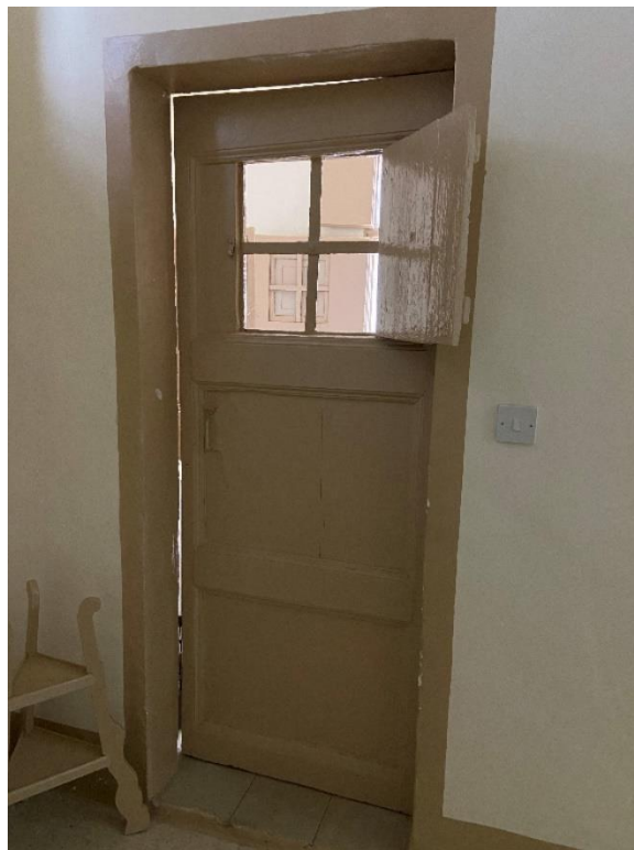
Figure 57. Door with peep window from the corridor into the correctional room.
