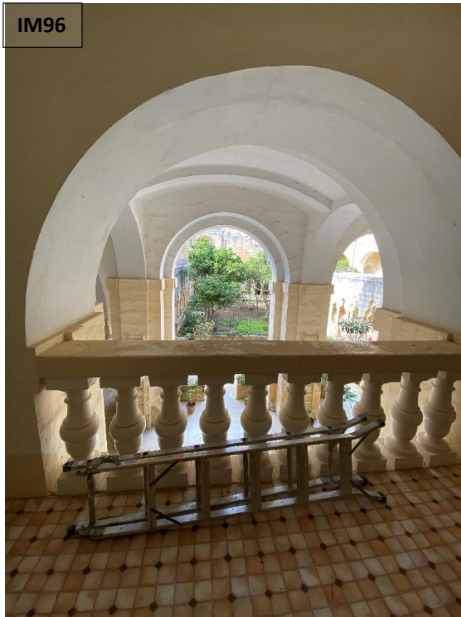
Details: Balustraded walkway overlooking the enclosed garden
