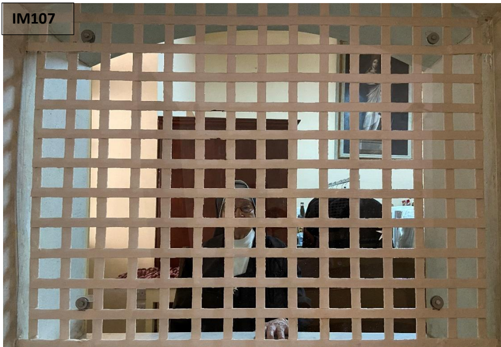
Grilled communication window
