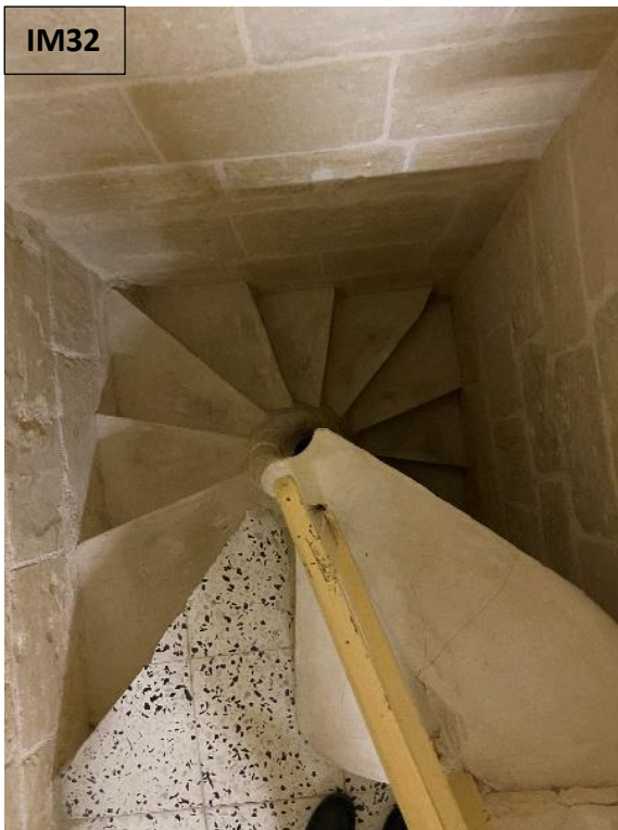
Spiral staircase joining lower and upper sacristy
