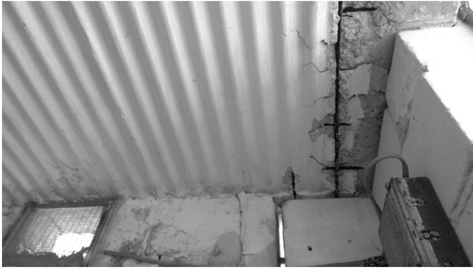
Figure D.32: Spalling of concrete roofs
