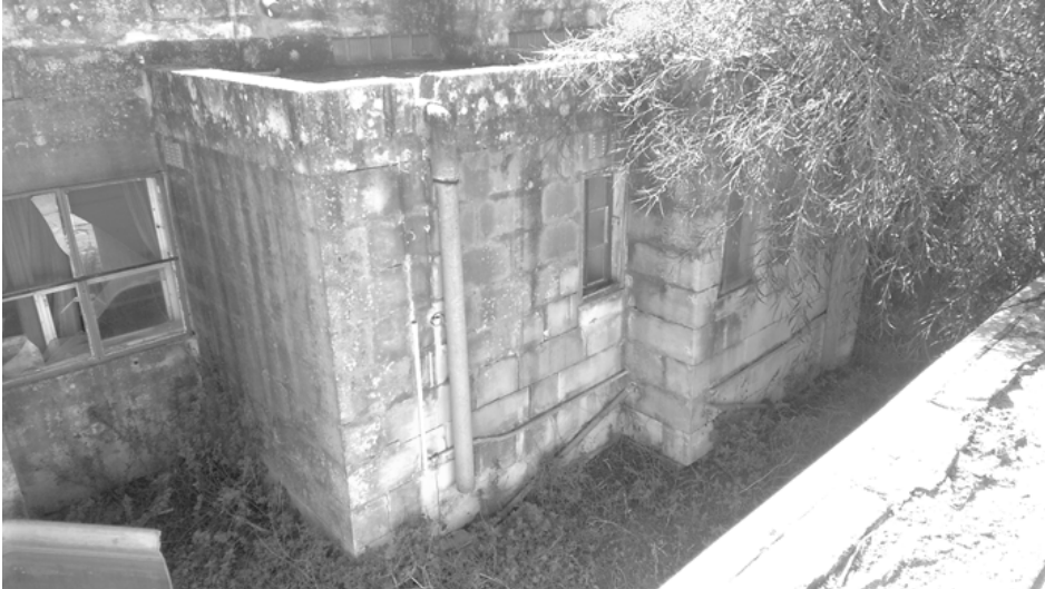
Figure D.37: Apertures with broken glass panes
