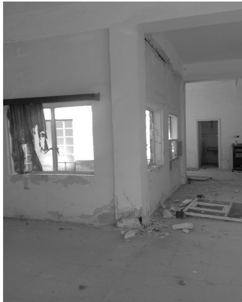
Figure D.31: Spalling reinforced concrete beams and columns
