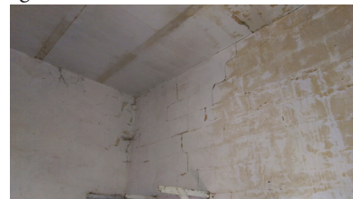
Figure D.29: Flaking paint on walls
