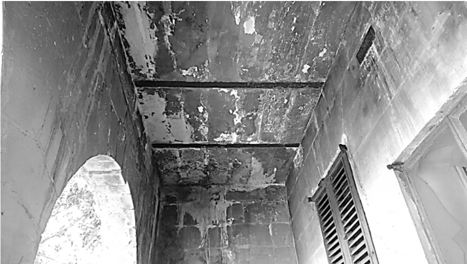
Figure D.35: Carbonised walls and ceilings
