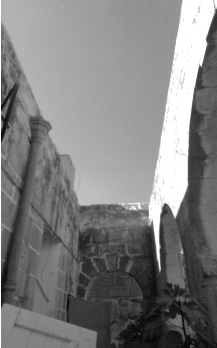
Figure D.34: Collapsed roof of portico
