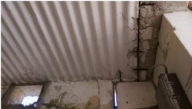
Figure D.34: Collapsed roof of portico
