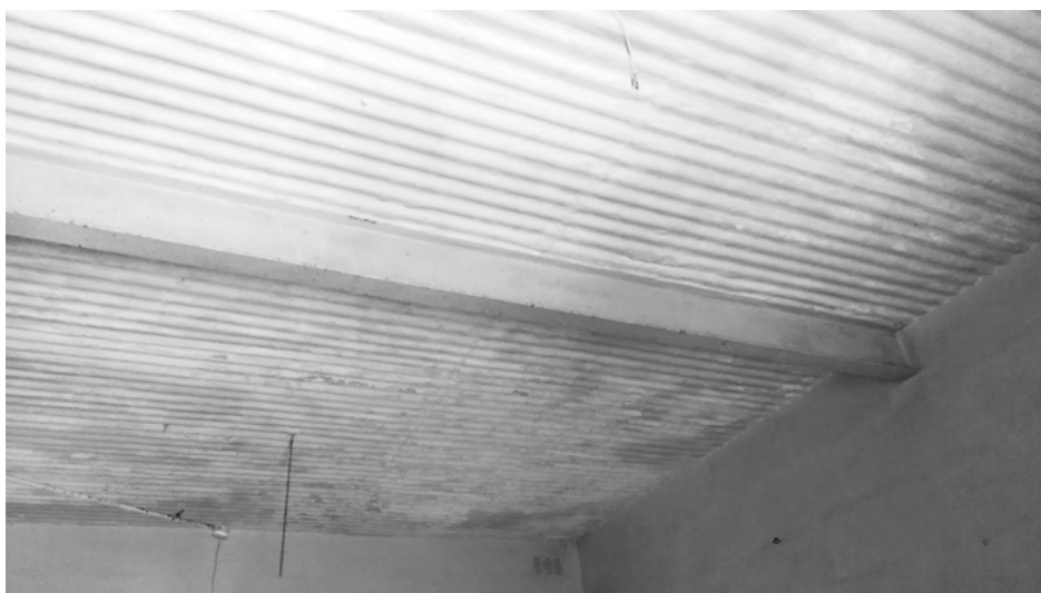
Figure D.24: Reinforced concrete roofs where corrugated metal sheets were used as formwork
