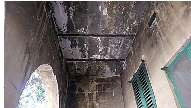
Figure D.36: Steel beams exposed to fire
