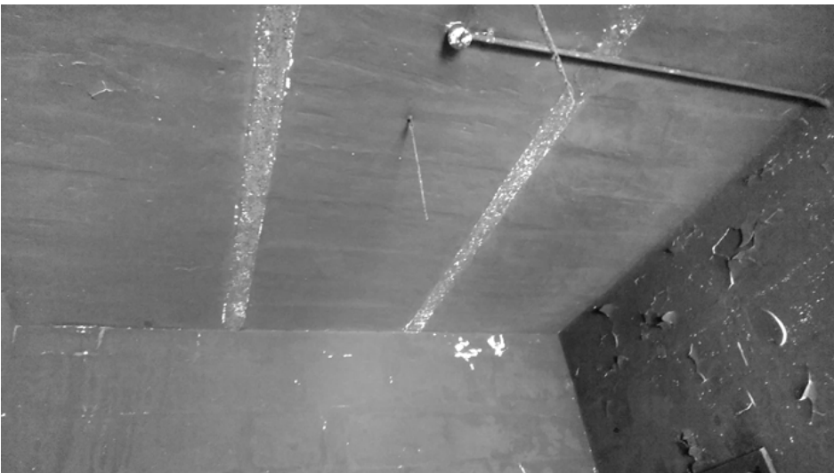
Figure D.36: Steel beams exposed to fire
