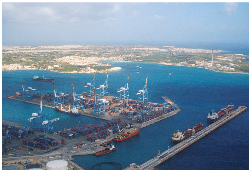
Marsaxlokk Bay is surrounded by development such as the Delimara Powerstation and Malta Freeport
