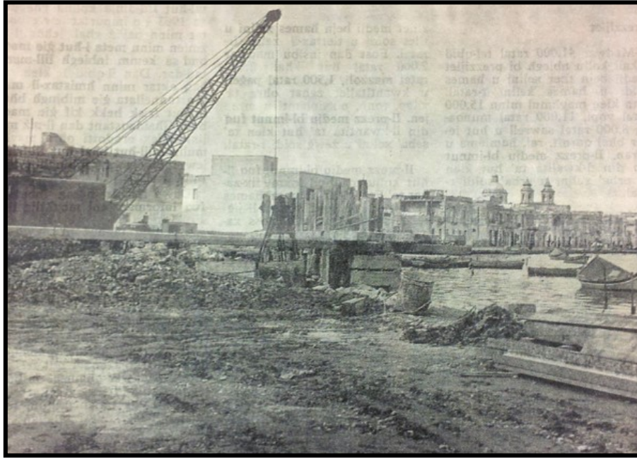
Picture 3: Works in progress at Marsaxlokk
