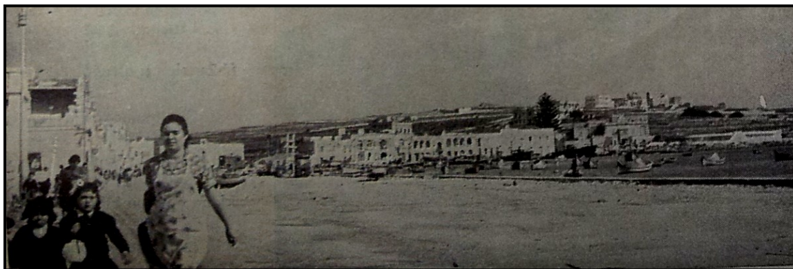
Picture 5: Marsaxlokk's 1,200 feet quay widened by circa 60 to 80 feet
