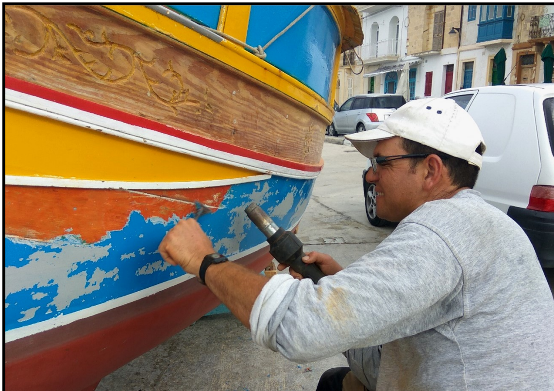
Picture 71: Burning and scraping off the layers of paint
