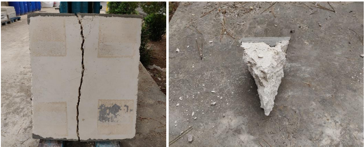
Figure F.14 – Left , failure mode front elevation; right , wedge cone failure
