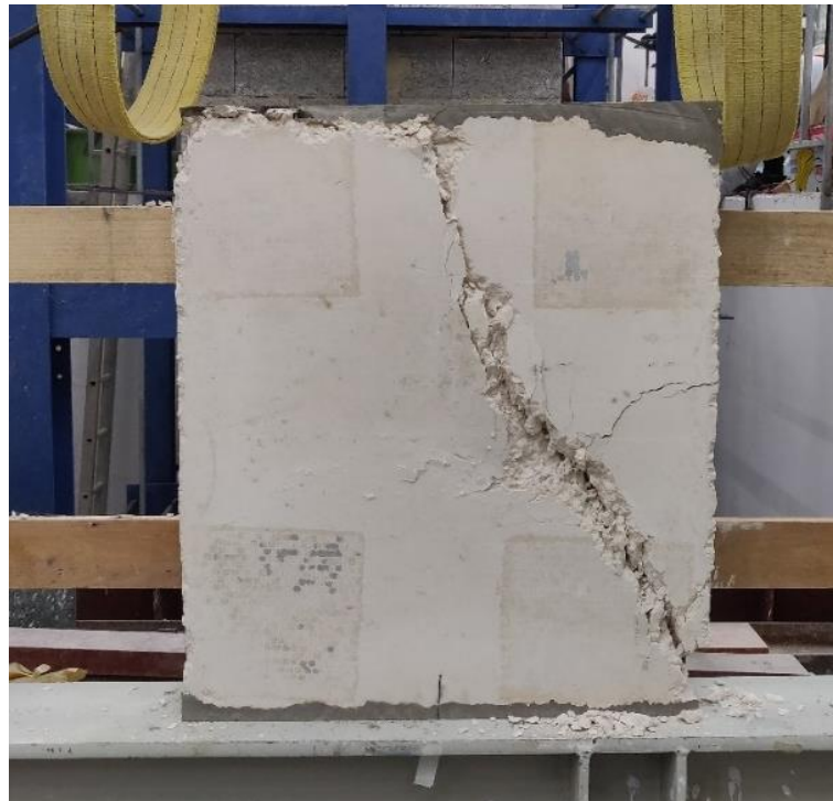
Figure 4.8 – Failure mode front elevation
