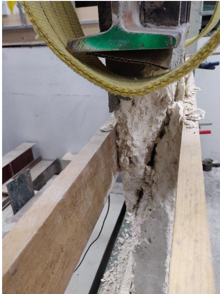
Figure F.4 – Diagonal crack failure mode for wall 1, setup 2
