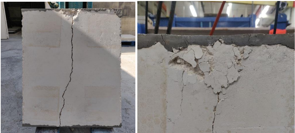
Figure F.16 – Left , failure mode front elevation; right , wedge cone failure
