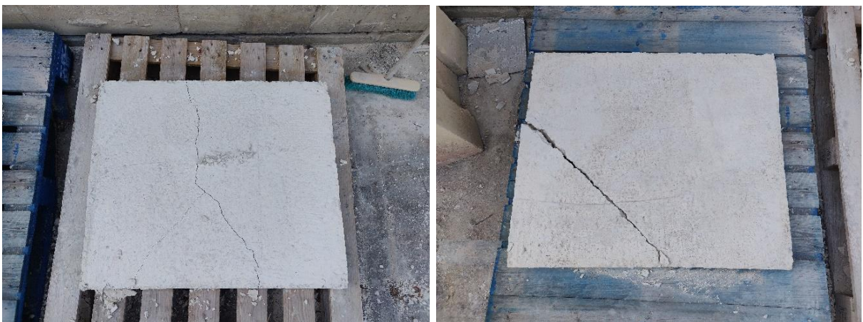
Figure 4.27 – Cracked walls which had to be abandoned
