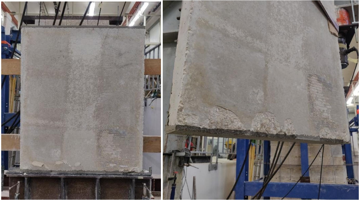
Figure 4.40 – Front elevation; spalling of concrete along the bottom edge
