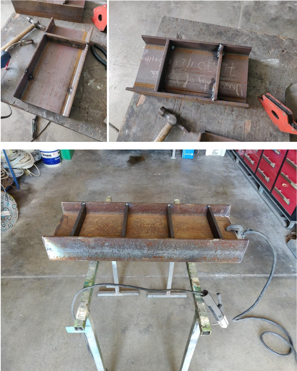
Figure G.1 – Manufacturing of the steel beams used for distributing the point loads
