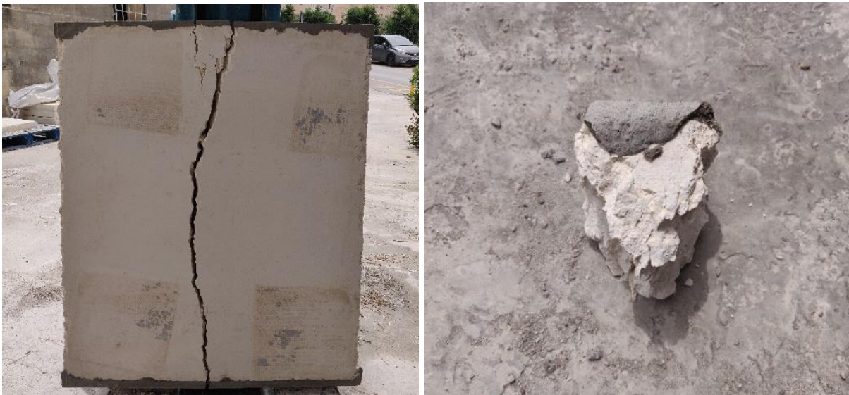
Figure F.12 – Left , failure mode front elevation; right , wedge cone failure
