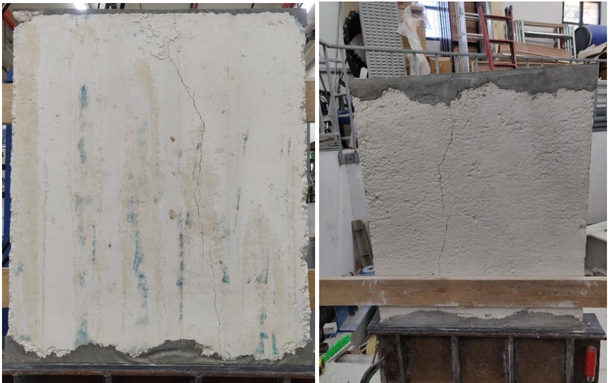
Figure 4.19 – Left , failure mode front elevation; right , failure mode back elevation
