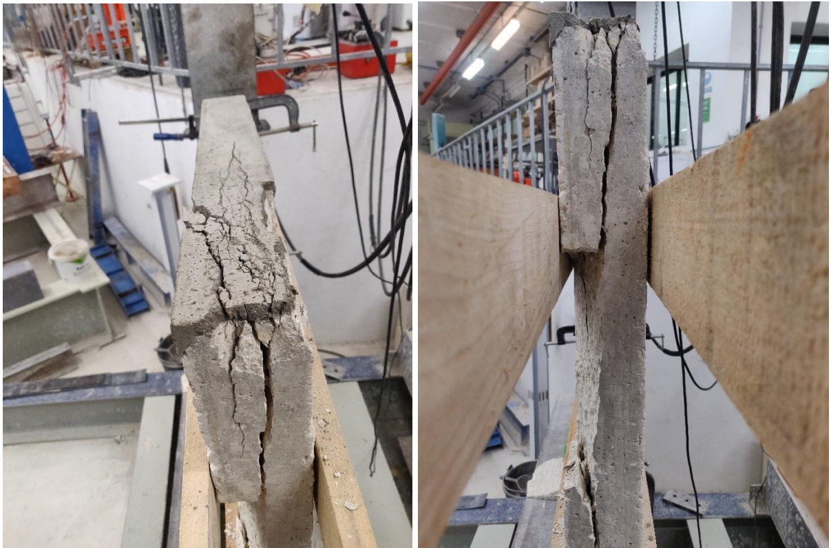
Figure 4.45 – Failure mode upon releasing the loads sequentially
