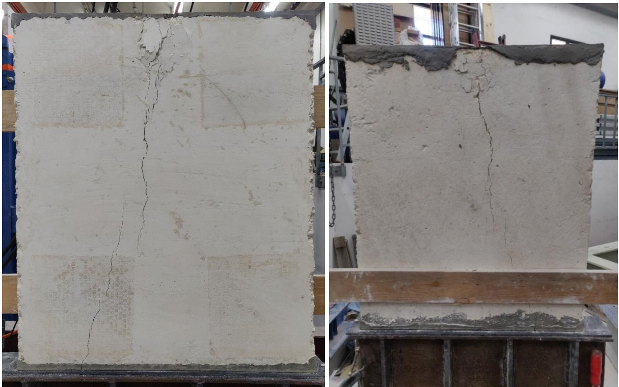
Figure 4.23 – Left , failure mode front elevation; right , failure mode back elevation
