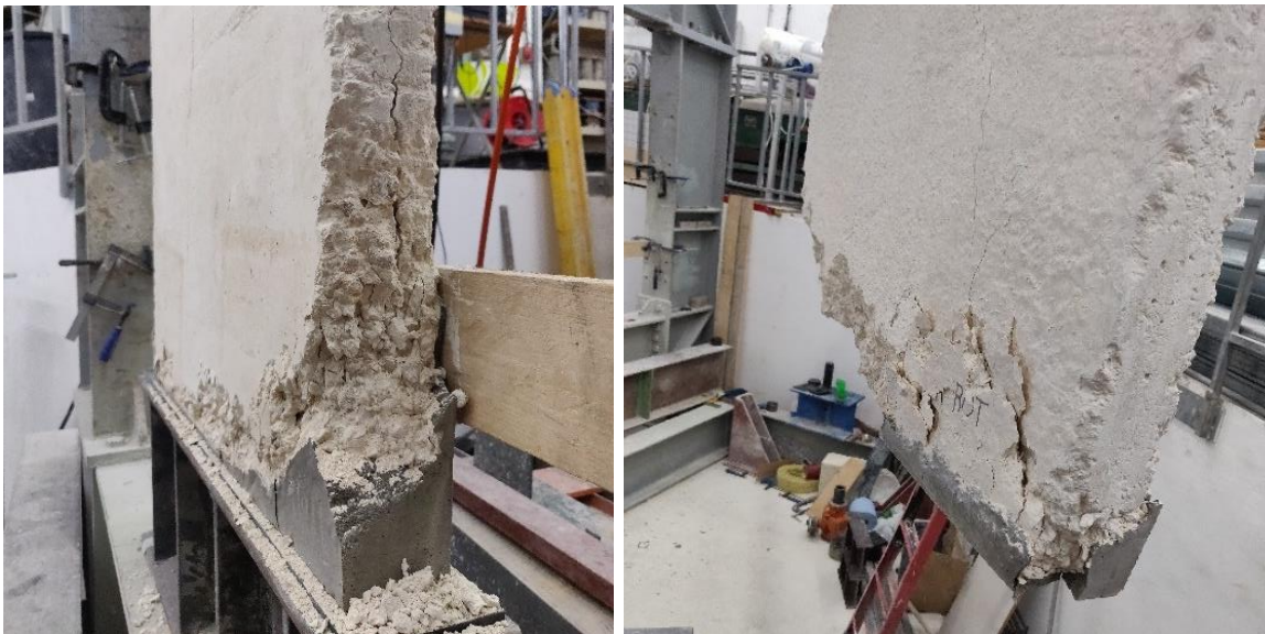
Figure F.26 – Crushing failure along the pre-damaged surface
