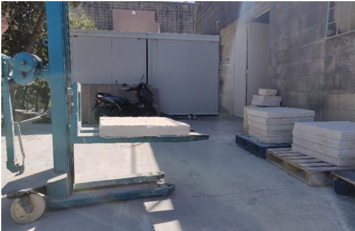
Figure 3.15 – Moving the wall from outside the laboratory using a forklift
