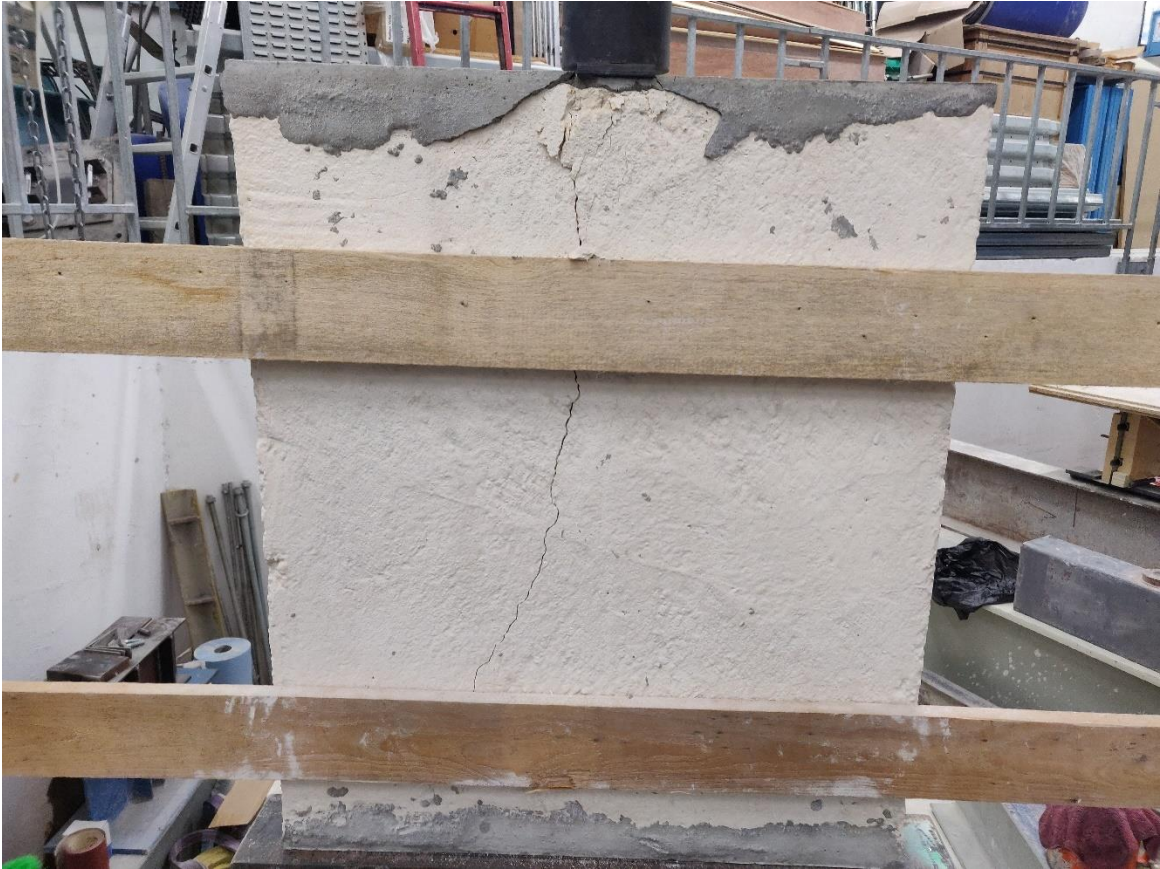
Figure F.9 – Failure mode back elevation
