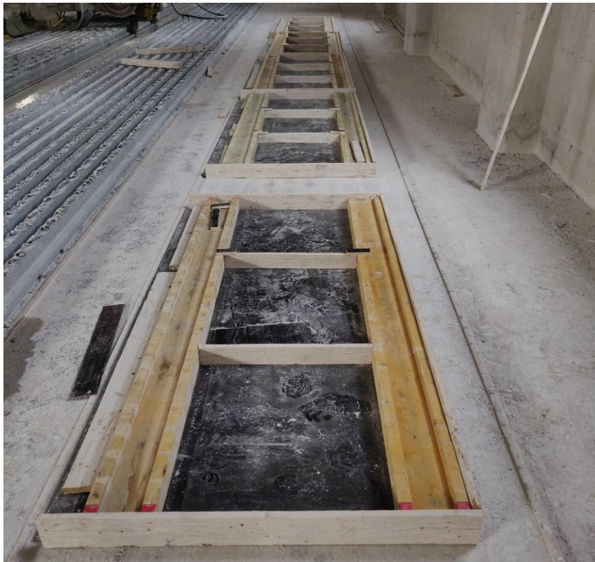
Figure 3.4 – Formwork setup before casting
