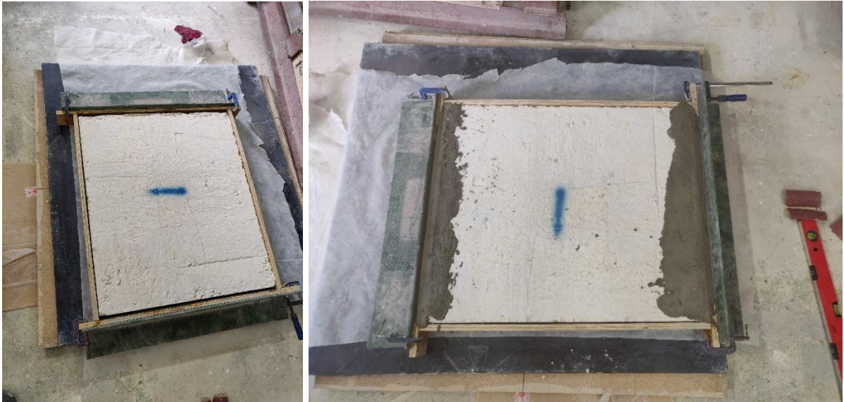
Figure 3.5 – Left , formwork for grouting; right , grouted Wall Panel
