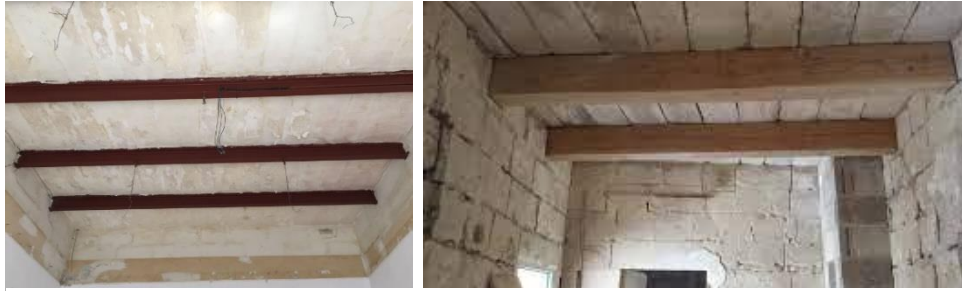
Figure 1.3: Xorok supported by steel or timber beams
