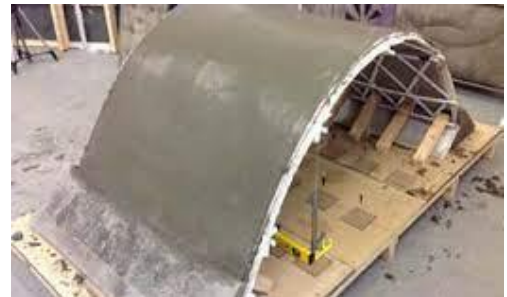
Figure 1.4: Formwork for a concrete shell
