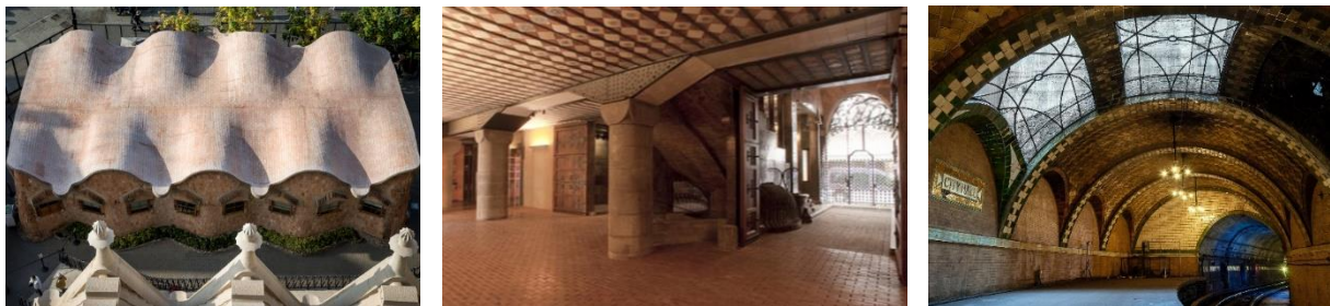
Figure 3.20: Left: The roof of the School of the Sagrada Familia; Middle: Coach house in Palau Güell Right: New York's City Hall Subway Station
