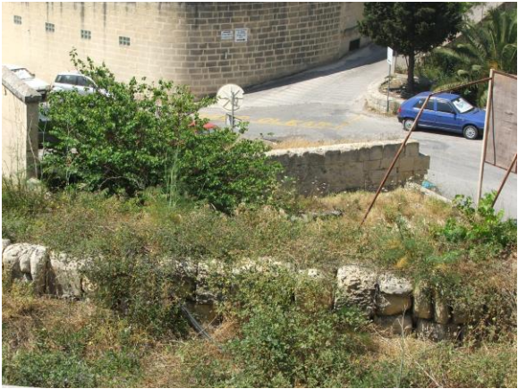
Sections of the plant infested parapet, probably missing some courses, broken stones, and pollution.
