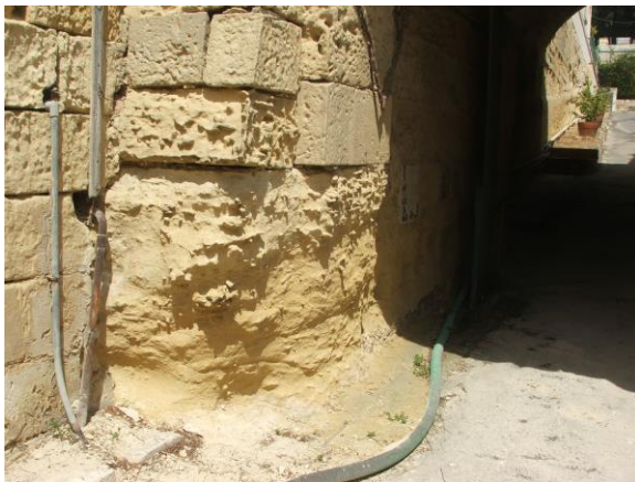
Alveolar erosion and tubular accretions.
