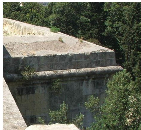
Figs. 52 and 53: Right flank, shoulder, cordon and parapet of St. Luke's Bastion. Very little deterioration but Lichen and algae growth and encrustation are more evident
