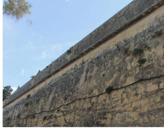
Fig. 13: The heavily encrusted right scarp.
