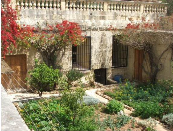
Underground stores and pump room.
