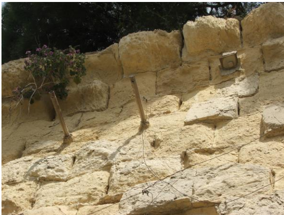
Eroded and broken masonry and accretions on curtain and cordon above the sally port.
