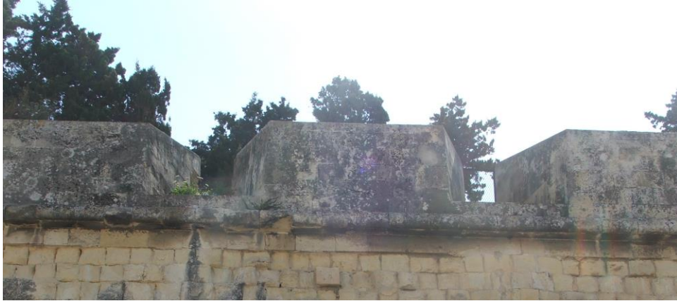
Fig. 23: Right embrasures heavily encrusted with lichens and algae.
