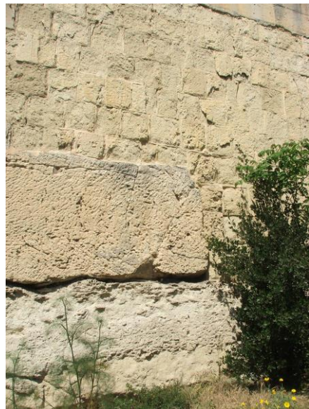
Fig. 46: Exfoliation and powdering.
