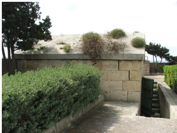
Fig. 36: Magazine with growth and open joints.
