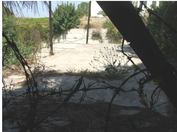
Metal staves and barbed wire on parapet.
