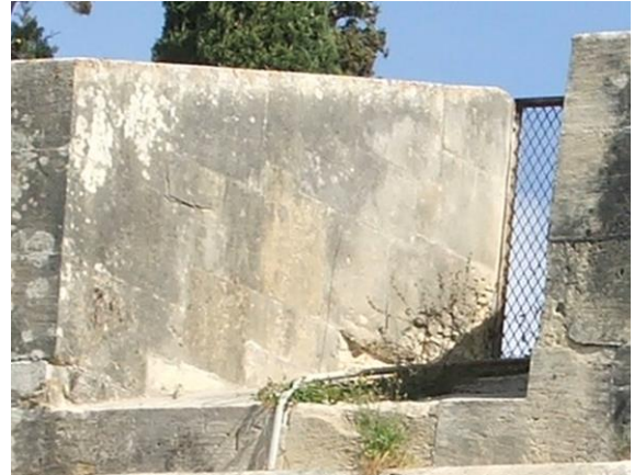
Fig. 21: Cheek of the second embrasure with as algae at upper and external levels and breakage.
