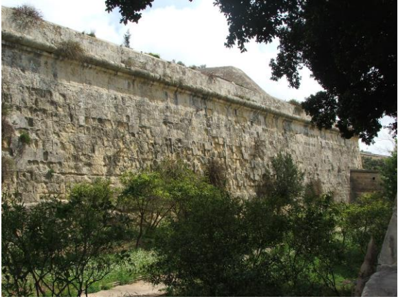
The right scarp – lower section more eroded.
