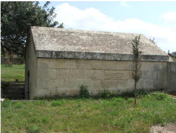
Alveolar erosion of the the right side.
