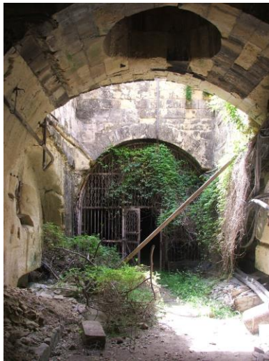
Aperture created in the ditch for the railway.
