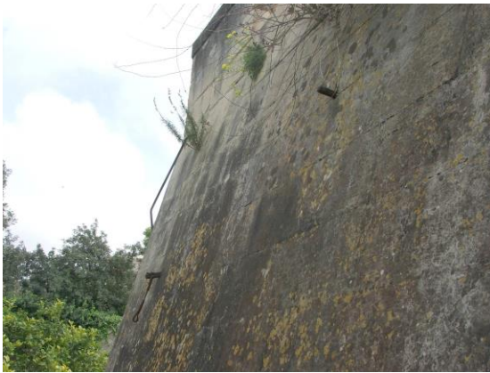
Fig. 40: Lichen, algae and accretions on left of counterscarp.
