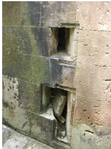
Fig. 42: Algae, lichen and breakage. Also signs of stone discolouration probably due to fires having been lit against the corner.
