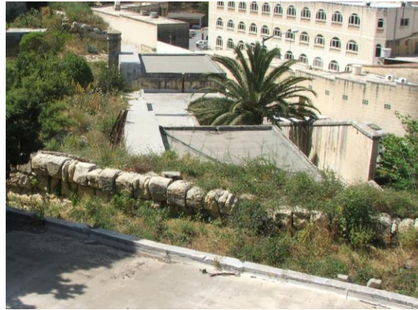
Sections of the plant infested parapet, probably missing some courses, broken stones, and pollution.
