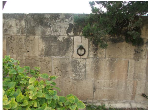
Fig. 14: Algae growth and encrustation within the parapet and gun-ring set in upper coralline limestone.
