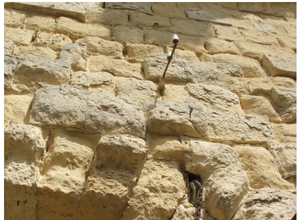
Eroded and broken masonry and accretions on curtain and cordon above the sally port.
