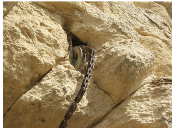
Gate's metal fittings and the powdering voussoirs.
