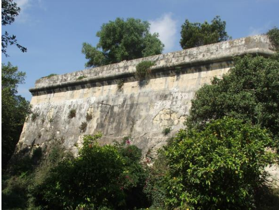
Flank with rendering from below cordon to rock.
