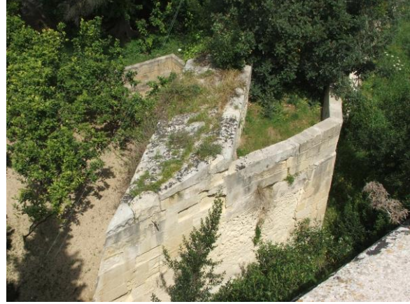
Close-up of the drop-ditch on the left.
