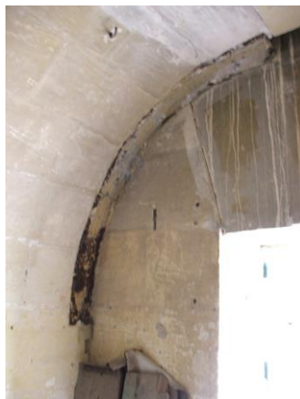
Fig. 38: Plant roots penetrating into magazine.
