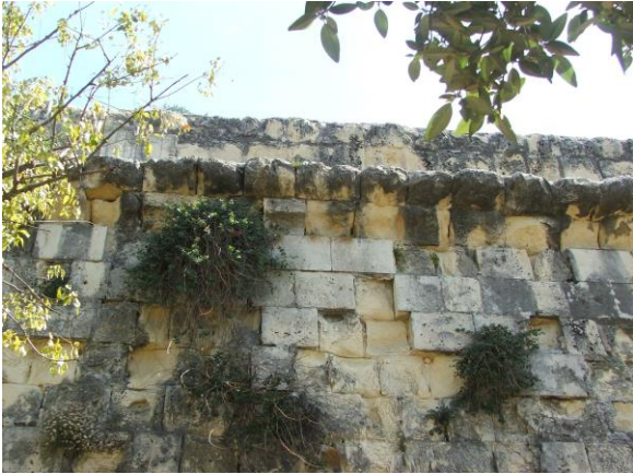
Deteriorated masonry, breakage, heavy black crust and plant growth on face, cordon and parapet.
