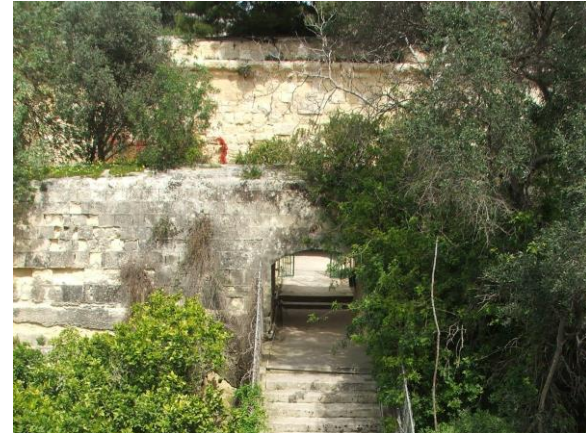
Broken stone, accretions, erosion, encrustation and growth on façade.
