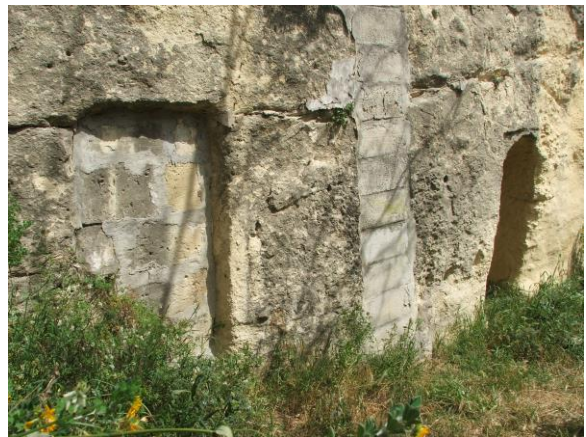
Excavations, trunking, cement and growth.
