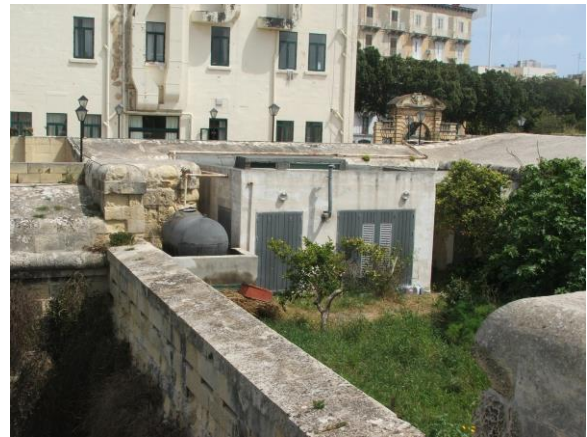
Eroded masonry and biological growth on loopholes. Accretions and extensions to the former utilities.
