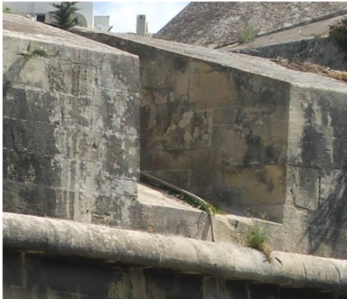
Fig. 20: Algae and lichen growth on parapet well as accretions and slight breakage.
