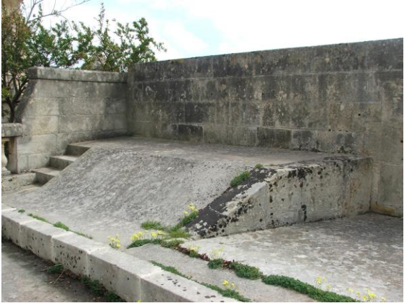
Figs 26 and 27: The banquette with heavy deposits of encrustation, algae, lichens and some growth.
