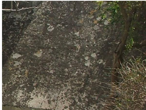
Fig. 31: Lichen and fungi on the internal slope.
