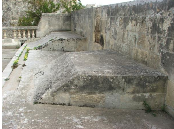
Figs 26 and 27: The banquette with heavy deposits of encrustation, algae, lichens and some growth.
