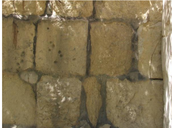
Cement pointing on the parapet's old fabric.
