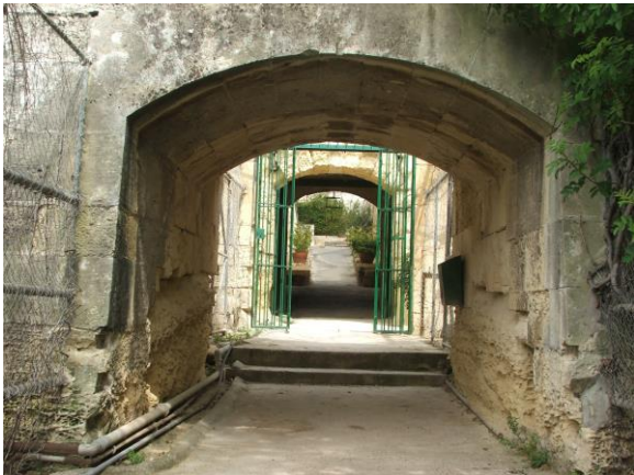
Broken stone, accretions, erosion, encrustation and growth on façade.
