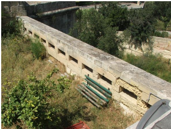
Eroded masonry and biological growth on loopholes. Accretions and extensions to the former utilities.
