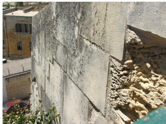
Fig. 25: Alveolar decay, black crust and growth on cheek.
