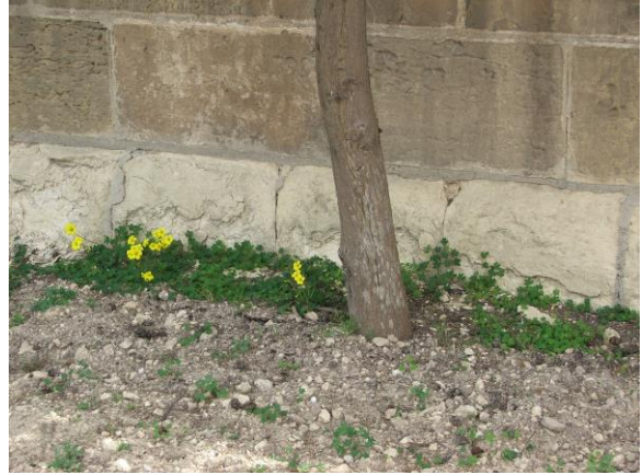
Fig. 16: The remains of the banquette and trees growing in such a delicate location.
