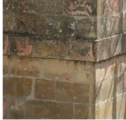
Figs. 34 and 35: Machinegun post structure showing Lichen, algae and fungal growth.
