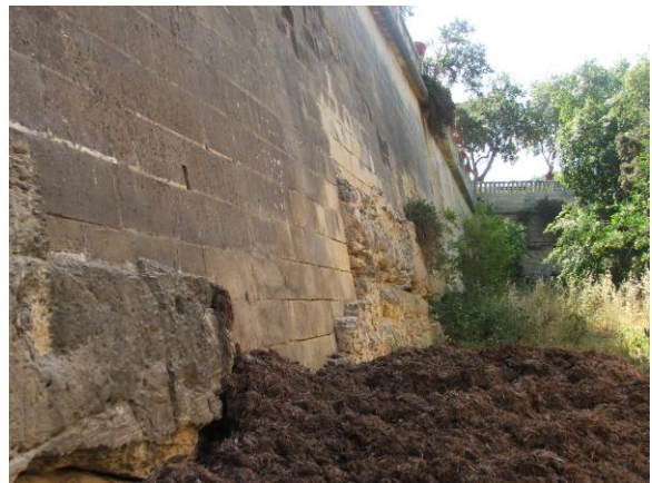
Manure pit in ditch near Triq Notre Dame .
