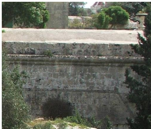
Figs. 52 and 53: Right flank, shoulder, cordon and parapet of St. Luke's Bastion. Very little deterioration but Lichen and algae growth and encrustation are more evident
