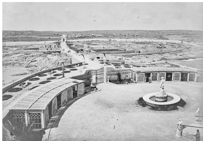
Figure 8. Photograph by Richard Ellis showing the access gate (top left) in the wall that enclosed the Dragonara Palace and the surrounding garigue grazing land. Late 19th century (reproduced by courtesy of the Richard Ellis Archive—Malta. M52-02).
