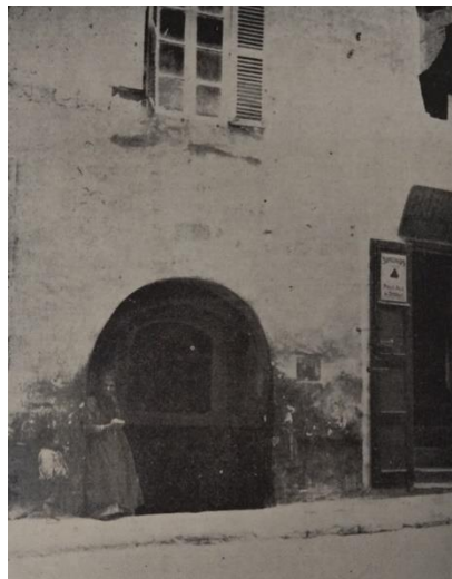
Fig. 24. Mina tač-Ċintura (Tunnel of Our Lady of the Girdle) (A. Critien)
