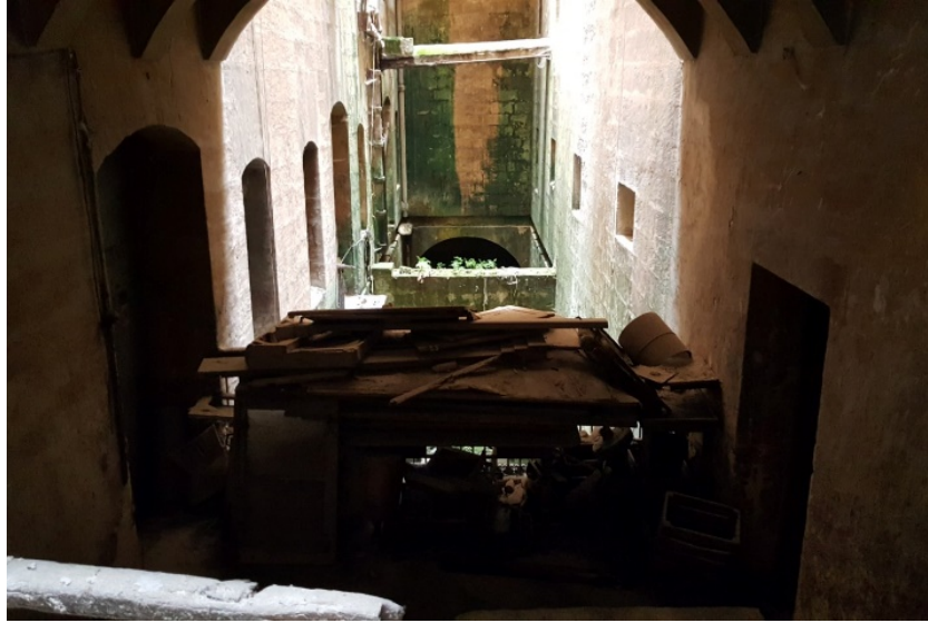
Fig. 67. View of the shaft as seen from one of the buildings.
