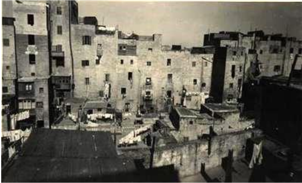
Photo 13. Washing hanging on rooftops of the Il-Mandraġġ and the rear of buildings along Marsamxett Road. (Jesmond Borg)
