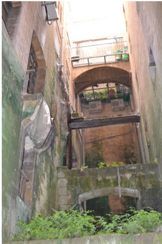
Fig. 68. The shaft from the opposite direction.
