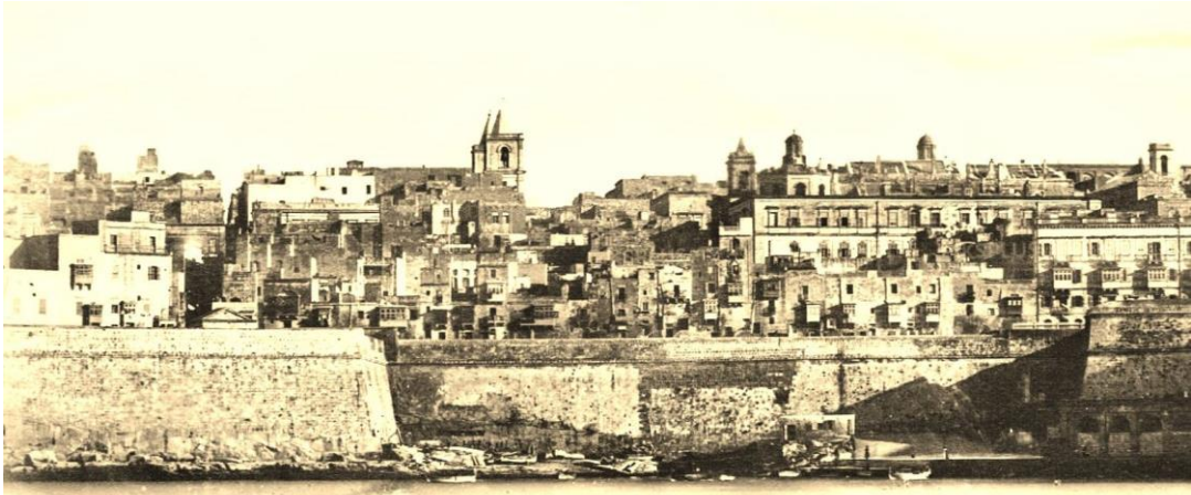
Photo 1. View of the Marsamxett Landing with the buildings of Marsamxett Road above the fortifications, c1895. (Anthony Bugeja)
