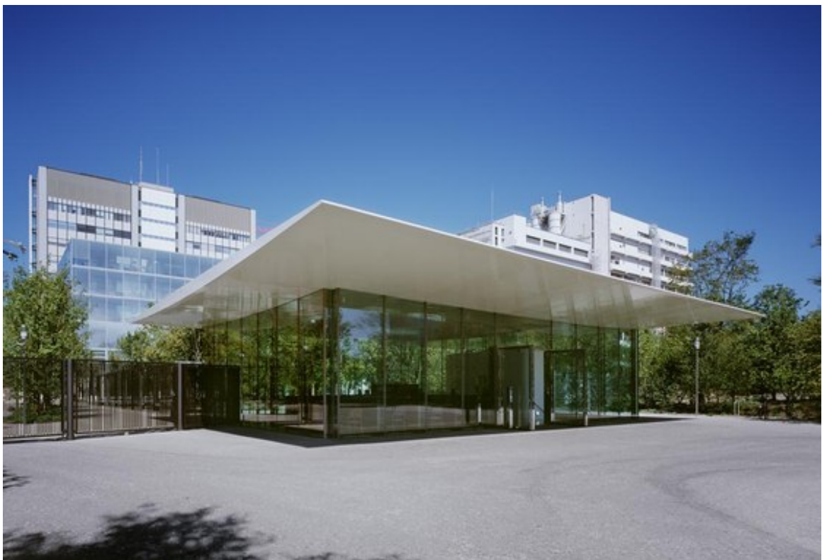
Figure 2-7: Novartis Campus Entrance Building, Basel, Switzerland. Roof is composed of GFRP sandwich panels (Roth, 2006)
