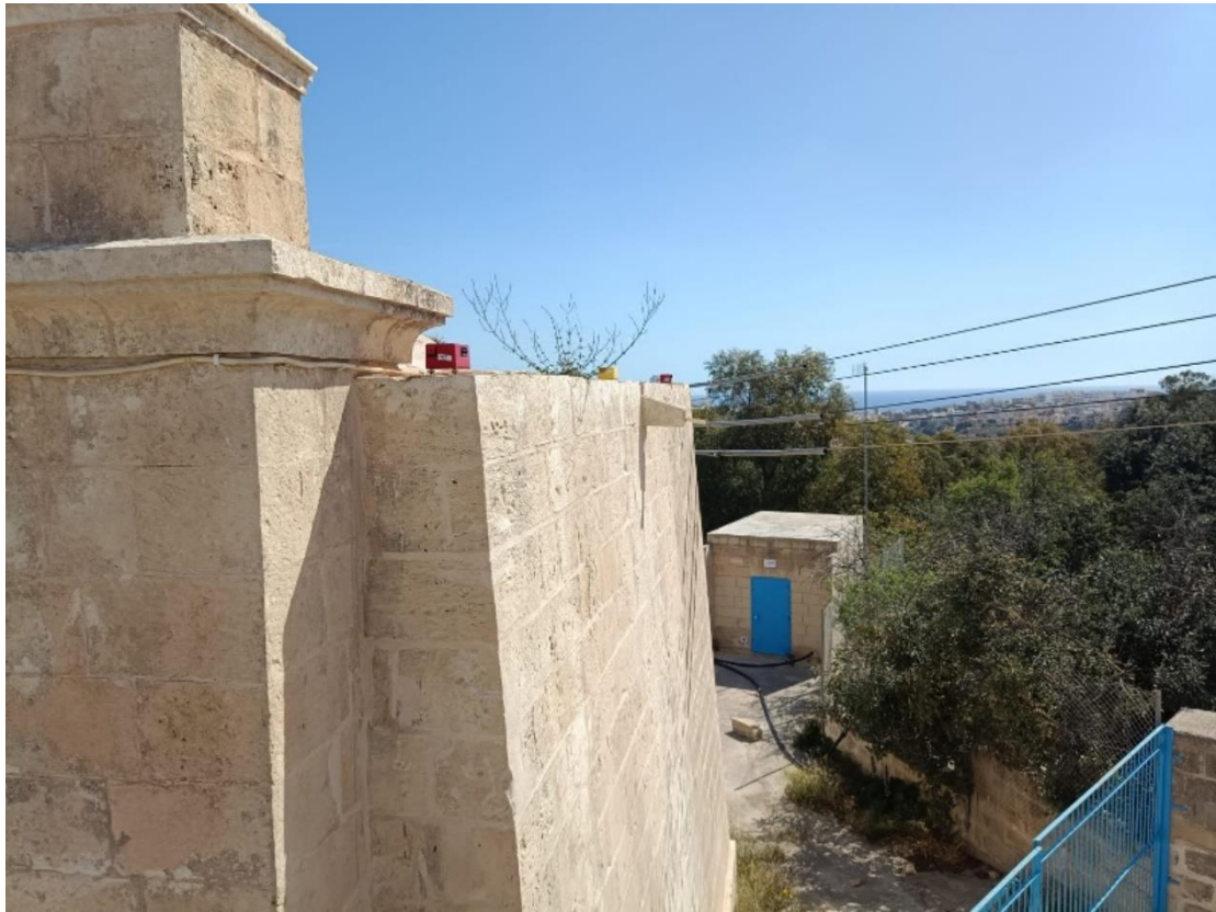
Figure 108 - Taking Reading on roof of chapel (Author, 06/05/2024).
