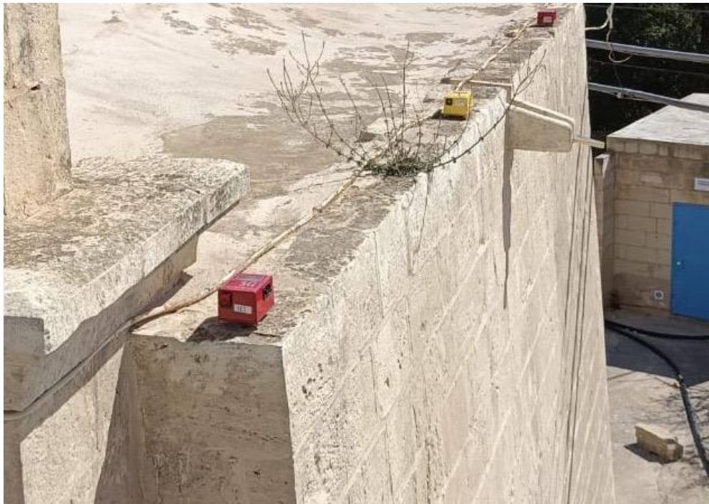
Figure 107 - Taking Reading on roof of chapel (Author, 06/05/2024).
