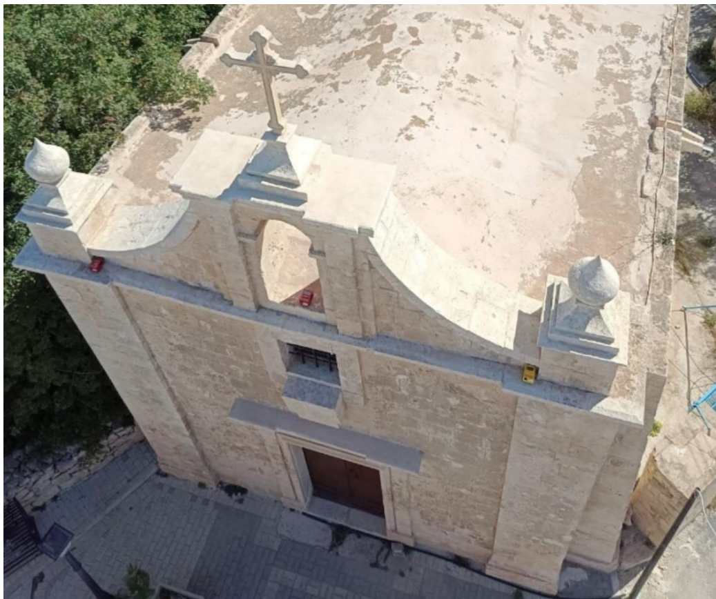
Figure 109 - Taking Reading on roof of chapel (Author, 06/05/2024).
