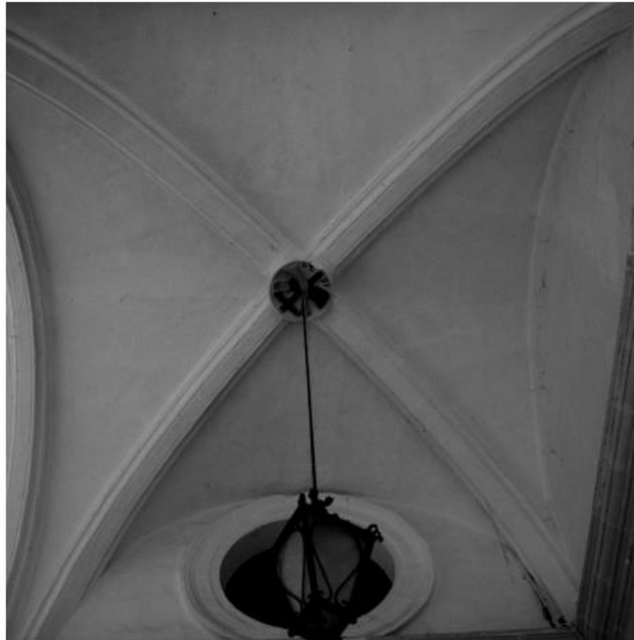
Figure A5 – Ribbed vault at Convent of Franciscan Minor Observants in Rabat, Malta. Reproduced from Galea (2016).
