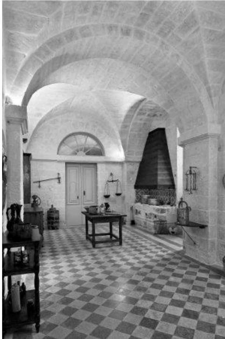
Figure A16 – Groin vaults of the kitchen at Carmelite Priory, Mdina.
