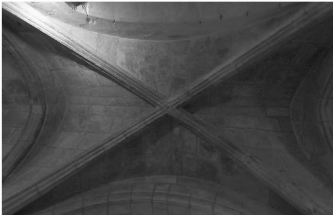
Figure A8 – Ribbed vault of Inquisitor's Palace, Birgu. Reproduced from Brincat (2020).
