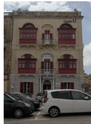
Photo CH6 - refurbished buildings
