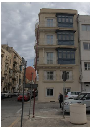
Photo CH7 - Refurbished buildings
