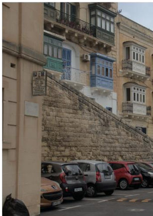
Photo CH4 - offset building, ruining view of residents behind and creating amorphous space
