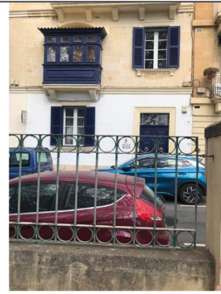
Photo CH3 - house with local features in well kept state
