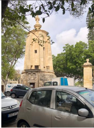
Photo AA1 - water tower across the street from Sarria chapel
