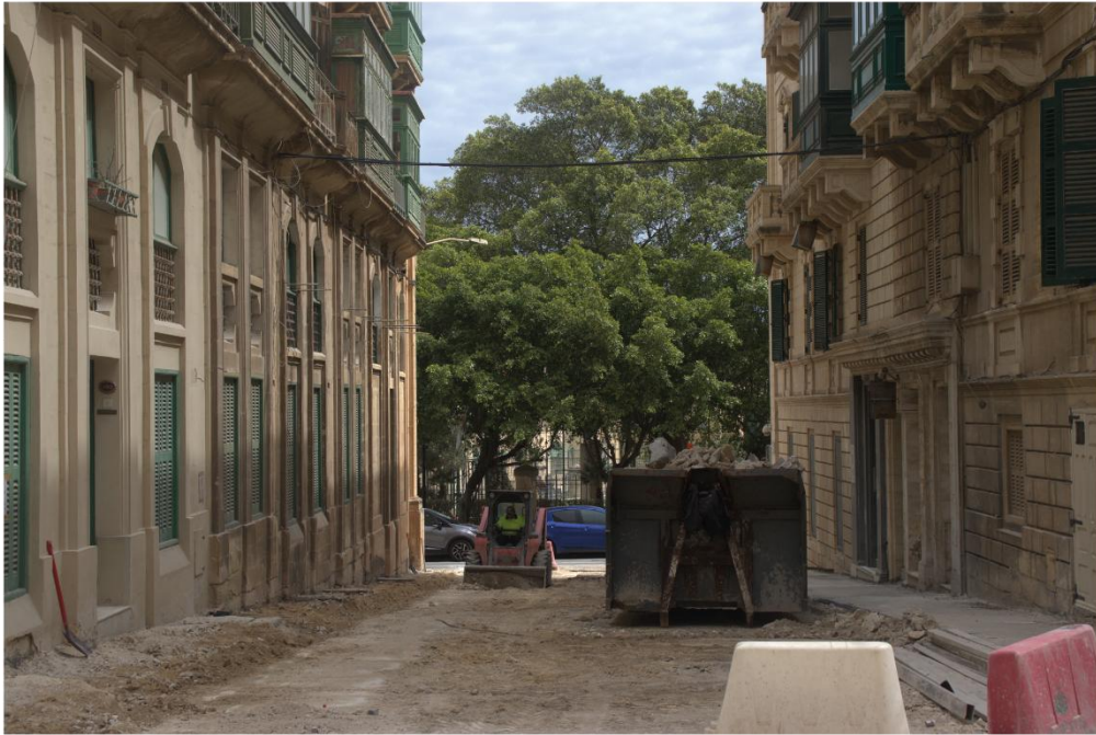
29 - Roadworks on Triq Macerata
