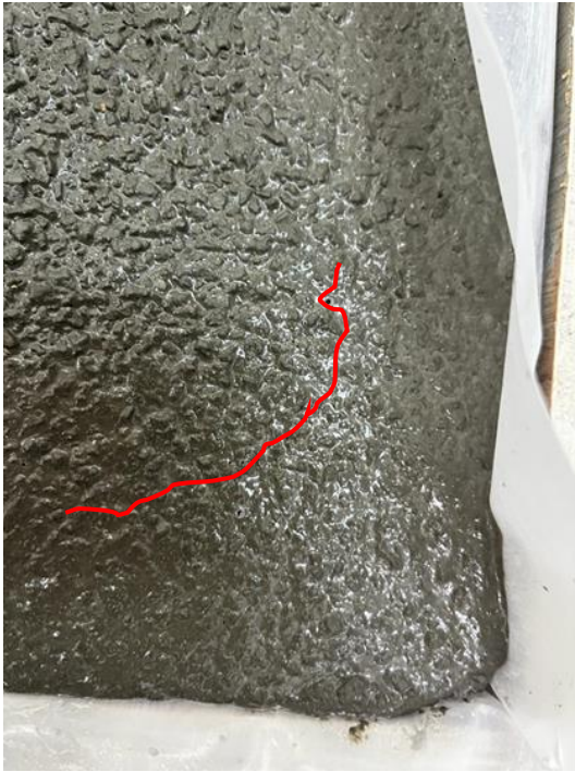
M0 - Control Mix – Visible Cracking
