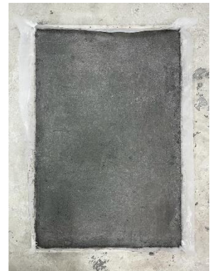
M0.5S – No Crack Formed
