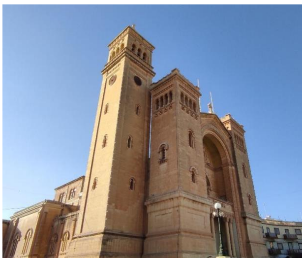
Figure 7: Parish Church of St. Peter in Chains
