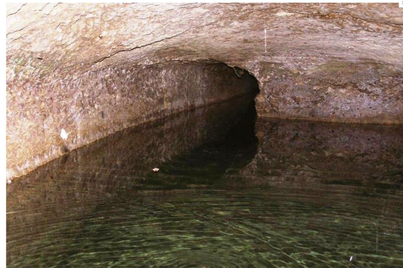
The Lunzjata perched aquifer gallery and its fronting water reservoir, located in the territory of Rabat, Malta. ©K.Buhagiar
