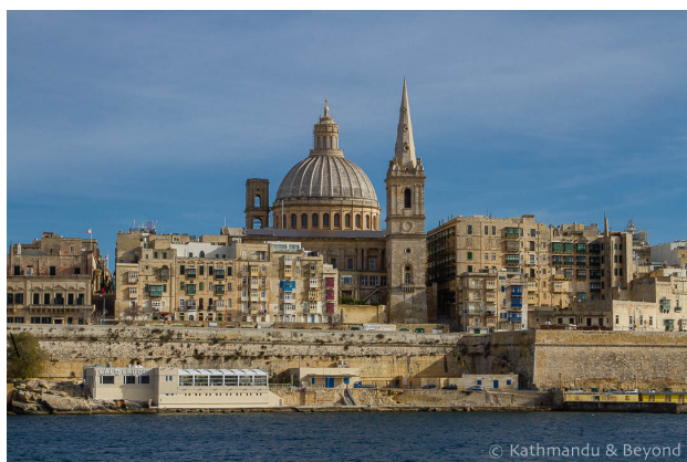
Figure 3 - St. Paul's Pro-Cathedral, built by the British to cater to the Anglican community in Malta, Via Kathmandu & Beyond, 2018
