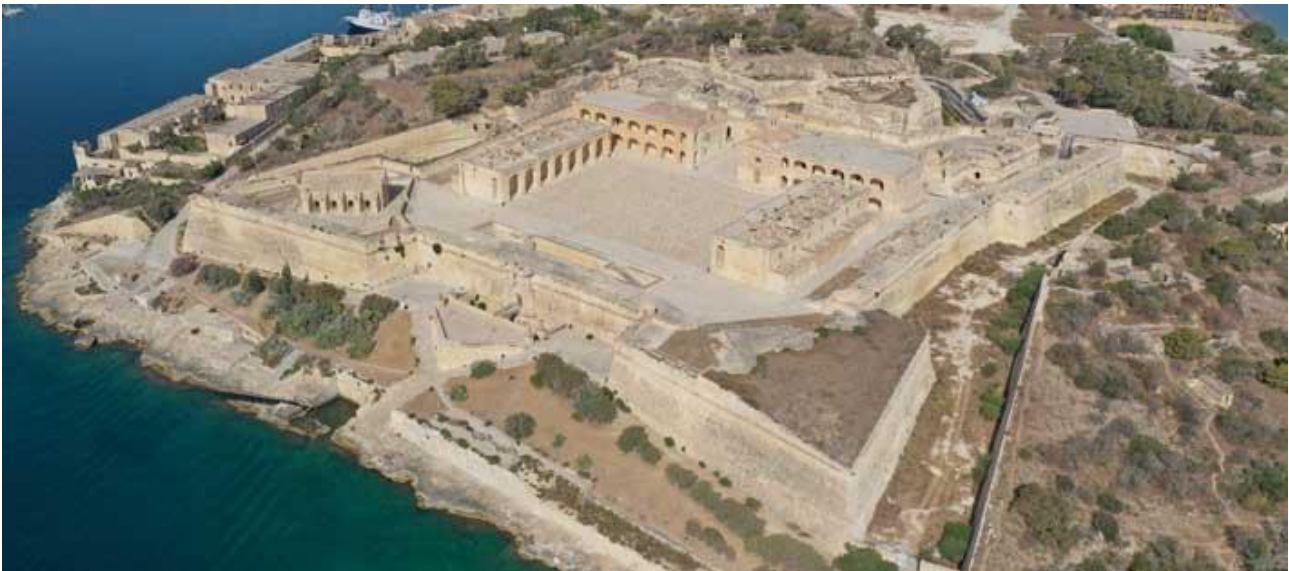
Figure 5 - Fort Manoel, Ariel view, Via The Malta Independent, 2023
