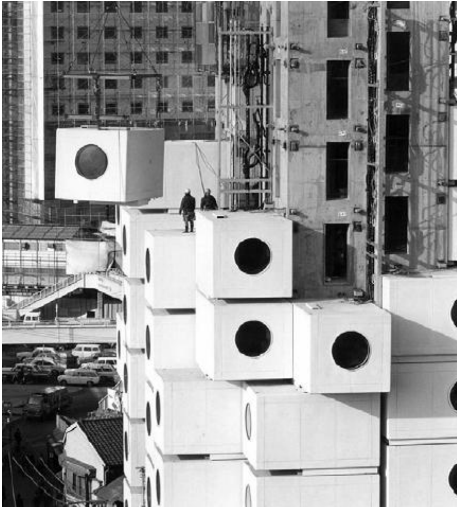
Figure 11 Metabolist Philosophy in Nakagin Capsule Tower - Modular Unit Installation (Minami, 2021)
