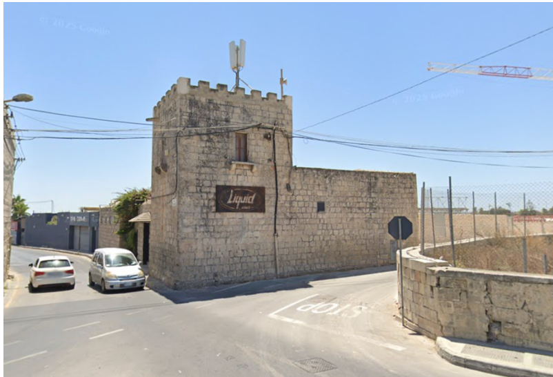
Figure A13 - Exterior of Liquid Club. Image source – Google Maps
