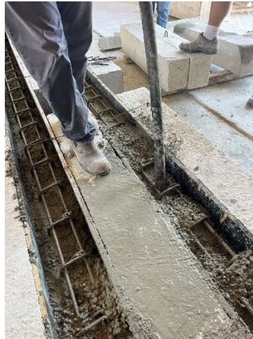
Figures 4.17, 4.18, and 4.19: Casting process / Vibrating of concrete / Addition of hooks for ease of transportation
