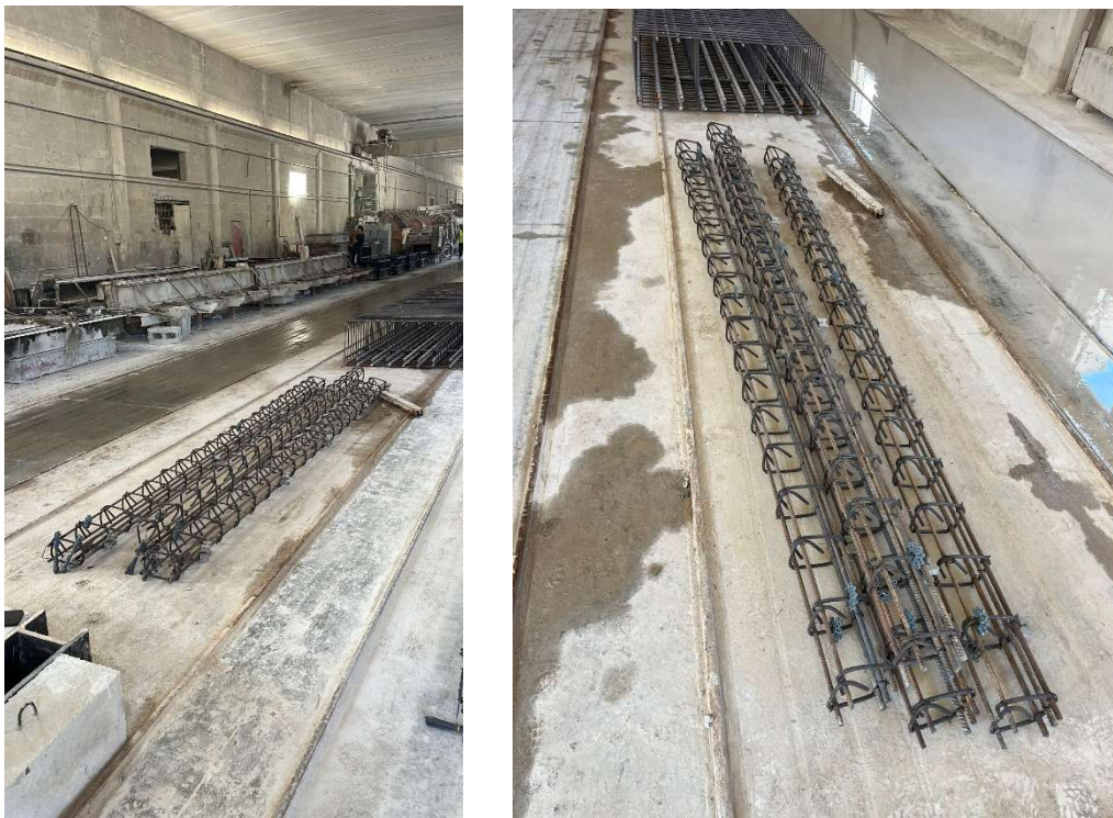
Figures 4.8 and 4.9: Beam reinforcement cages laid out on-site
