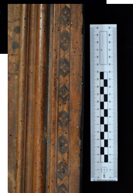
Fig. 94. Recovered 15th century frames that had been reused as repair material. The frames, manufactured out of solid walnut feature a central 'toppo' technique inlay banding.
