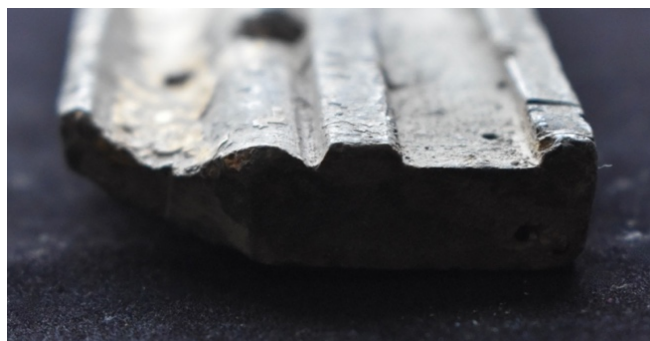
Fig. 61. Profile of original lower-tier frieze frame. (James Saliba, 2024)
