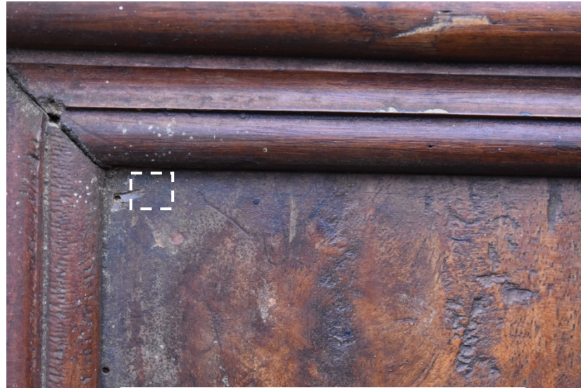
Fig. 40. - Area of sample lifting
