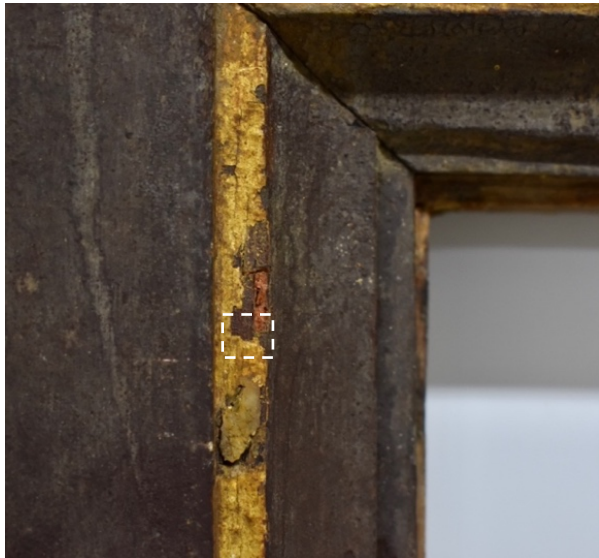
Fig. 32. - Area of sample lifting
