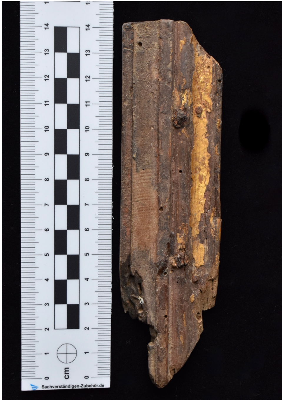
Fig. 60. Original lower-tier frieze frame with slot for toppo technique inlay banding. (James Saliba 2024)
