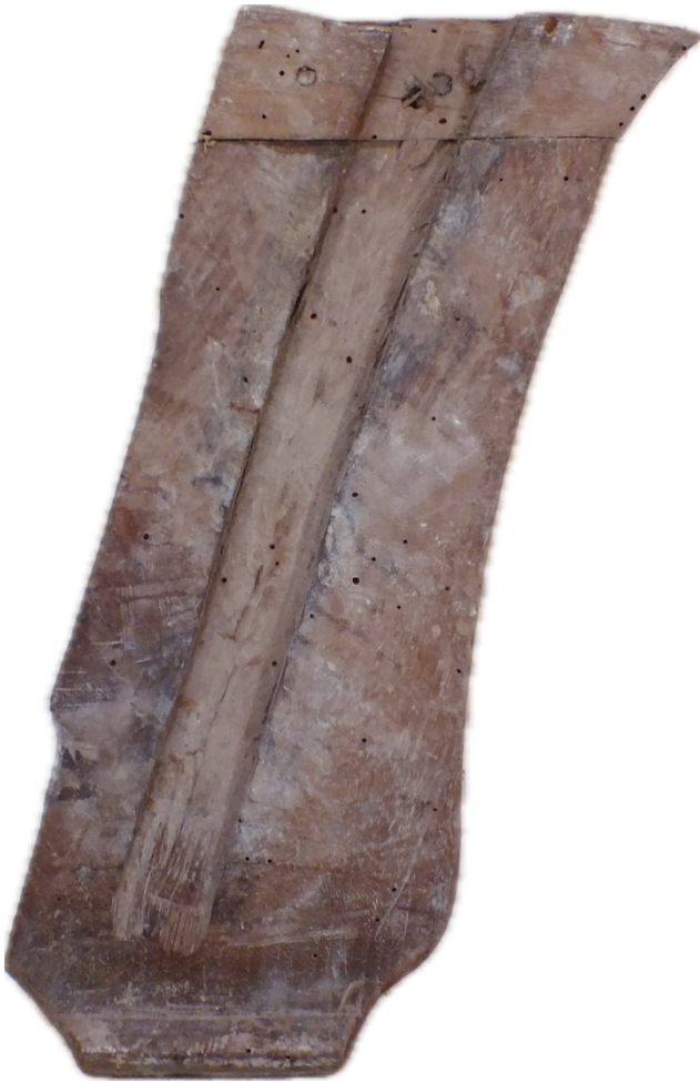
Fig. 77. Bottom side of armrest F.1.9 , revealing joinery groove for the attachment of stall side originally set at an 18-degree angle to the vertical axis. (conservation records: James Saliba, Bruno Ambrosio, 2016)
