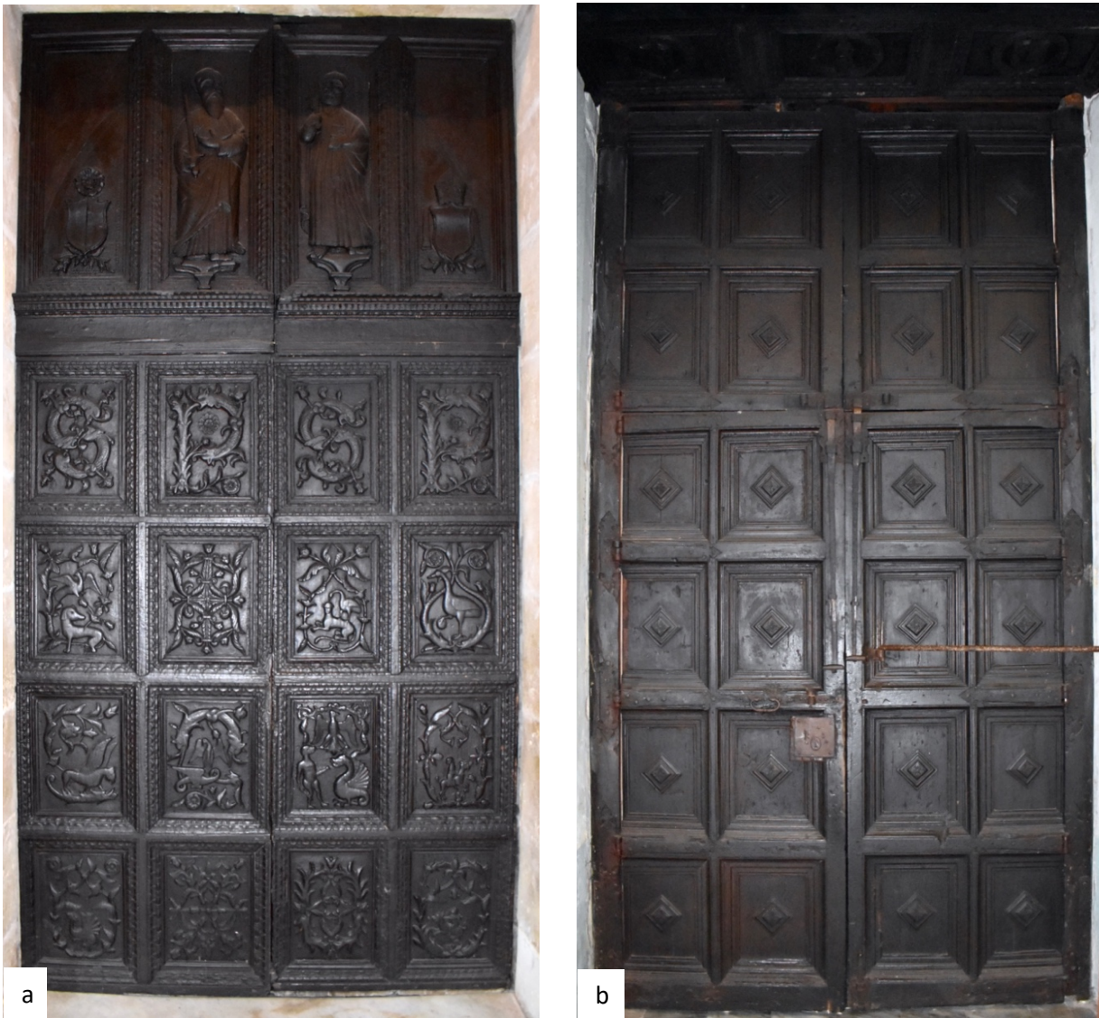
Fig. 3. The west door carved in chestnut by Cola Curmi and Johanni Calleja and installed as the main portal in 1535, later repurposed and currently serving as the door leading to the sacristy.
