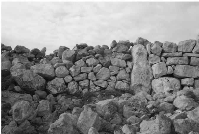
Figure 2.4. One of the megaliths embedded in a rubble wall at Borg in-Nadur (source: the author).
