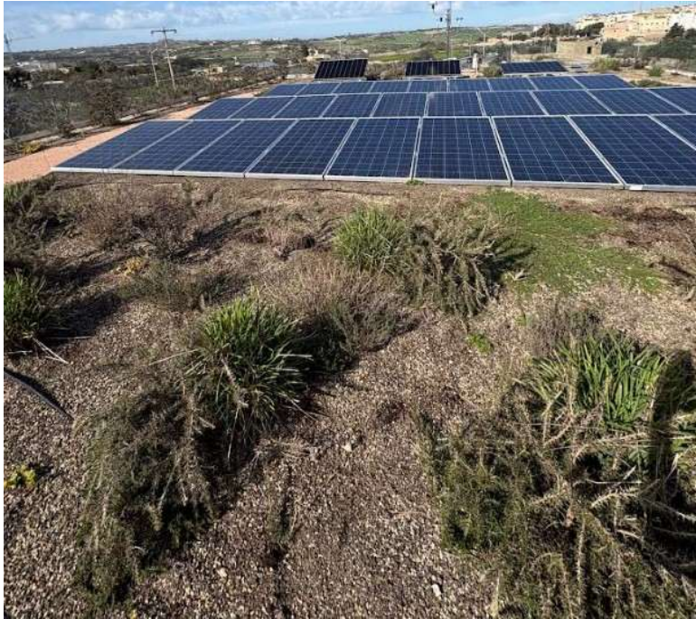
Figure 2. Green roof in Ghajn Water Conservation Centre, in Rabat Malta. Characterised by approximately 3000 plants featuring differing rates of retention and unique characteristics that make them suitable for Malta's arid climate. Additionally, this green roof also hosts photovoltaic panels for solar energy harvest
