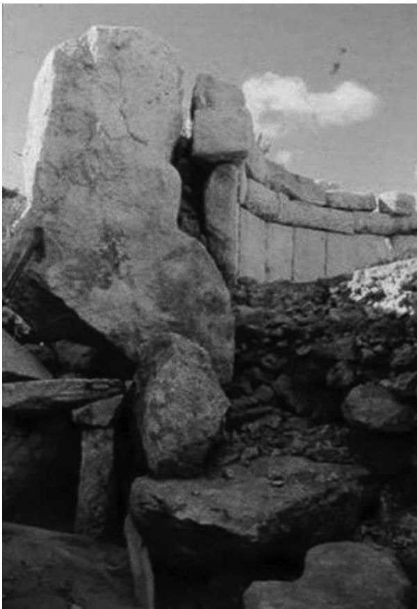
Figure 1. The collapse that occurred at Mnajdra in 1994.
