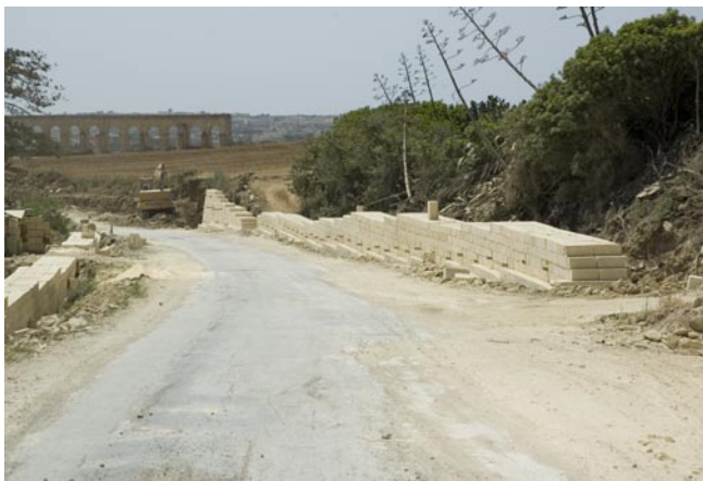
Works in progress on the Victoria-San Lawrenz road.
