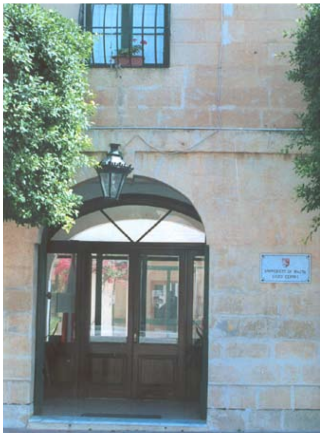
The premises of the University Gozo Centre is a 19th century building, and therefore requires ongoing attention.
