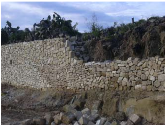
Rubble walls under re-construction.
