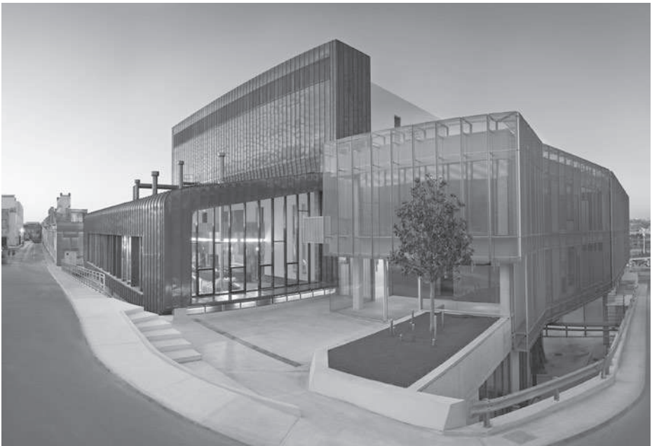
The state-of-the-art new brewhouse, inaugurated in September 2012.
