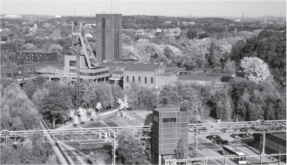
Figure 1. The Zollverein industrial complex in Land Nordrhein-Westfalen, Germany.
