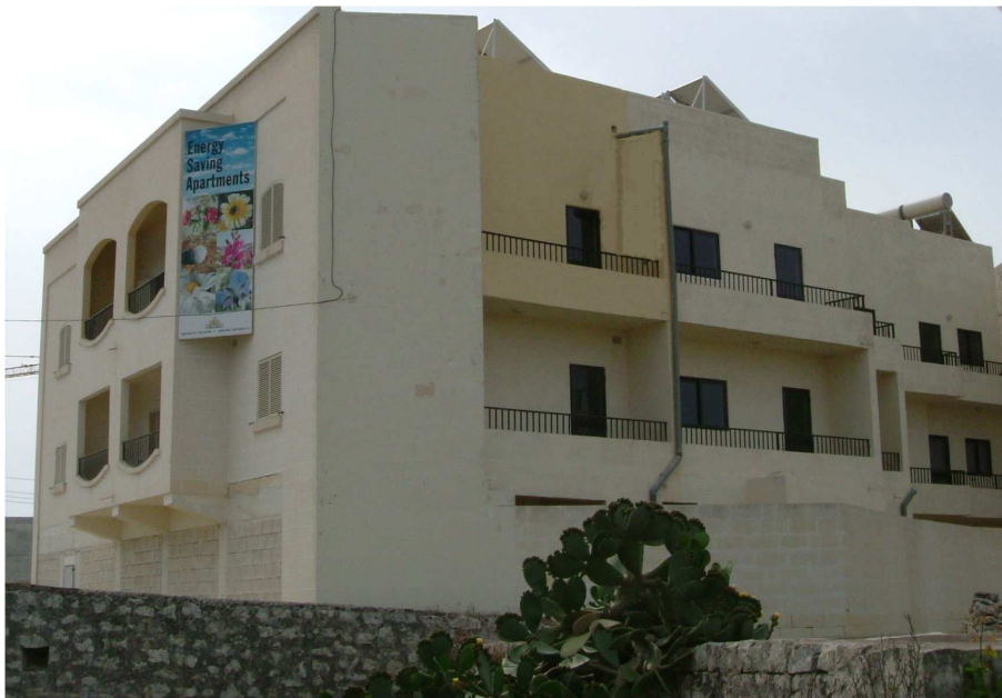
Figure 1: Tal-Ftieh Energy Efficient Housing Project, B’Kara-Malta, showing the northern and western facades, the latter with solar shading devices in the form of fin walls. A grid-connected 1.5 kWp PV system and twinned solar water heaters are also partly visible on the roof.
