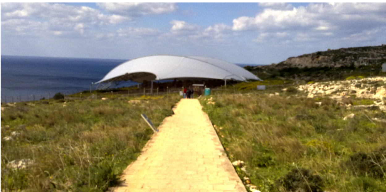
Figure 7.6: The recently finished shelter for the protection and preservation of the Mnajdra Temples; a similar shelter has been constructed for Hagar Qim Temples (George Cassar).
