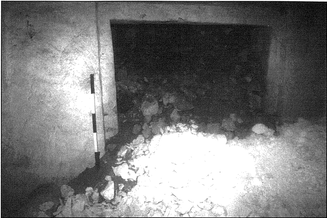
Plate 1: Original entrance containing soil below globigerina chippings
