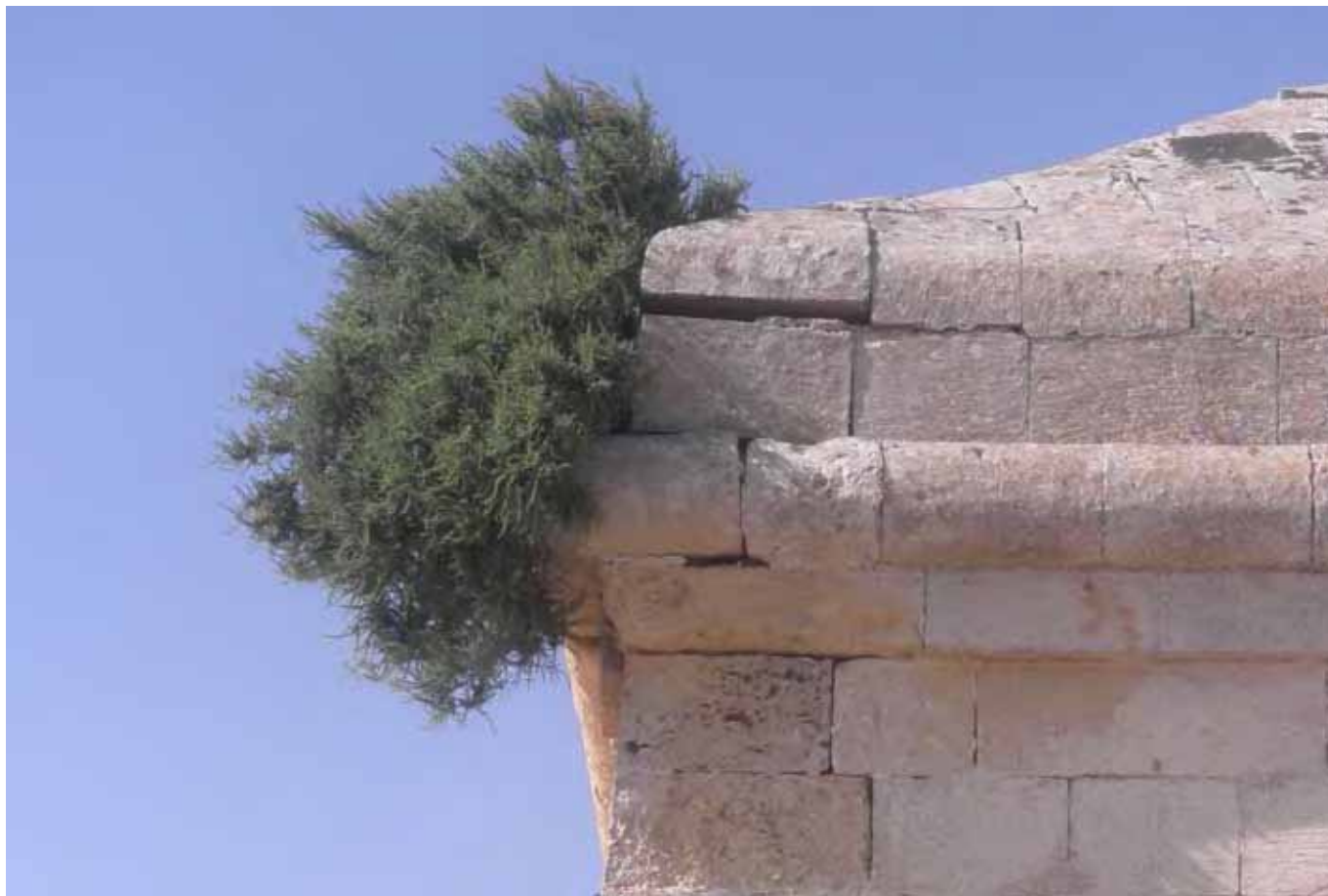
A salt tree shrub atop the parapet wall of St John's Cavalier. Note the dislodged masonry.
