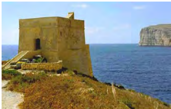
Xlendi Tower. (Photo courtesy of http://dinlarthelwa.org )
