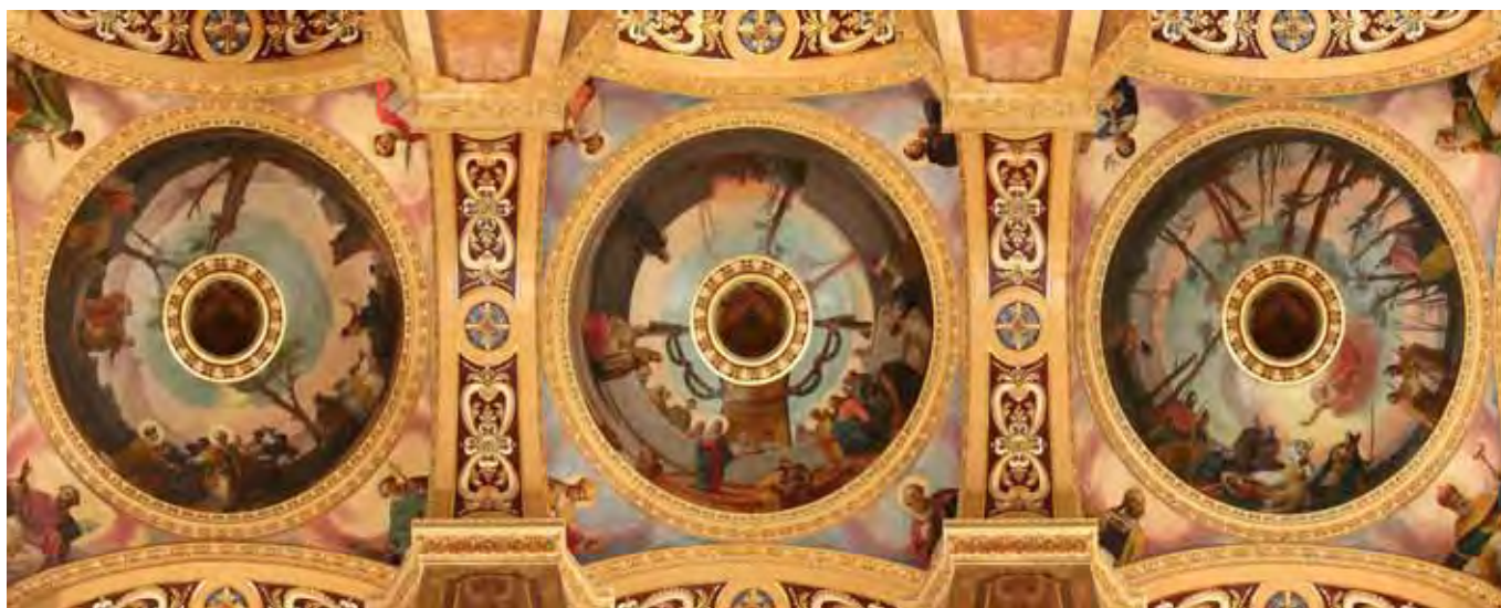
The recently-restored small domes and lunettes in the left apse (Virginio Monti).
