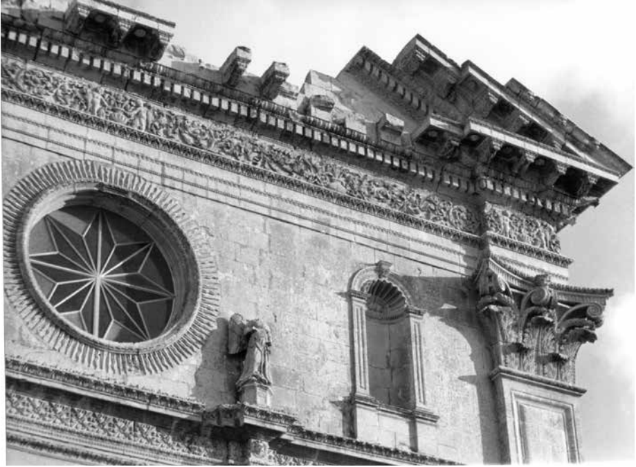
Fig. 13: Façade detail, old parish church, Birkirkara (Photo credit: Carmel Psaila)
