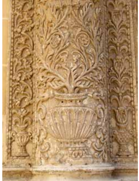
Fig. 7: Decorative detail of column, Attard parish church
