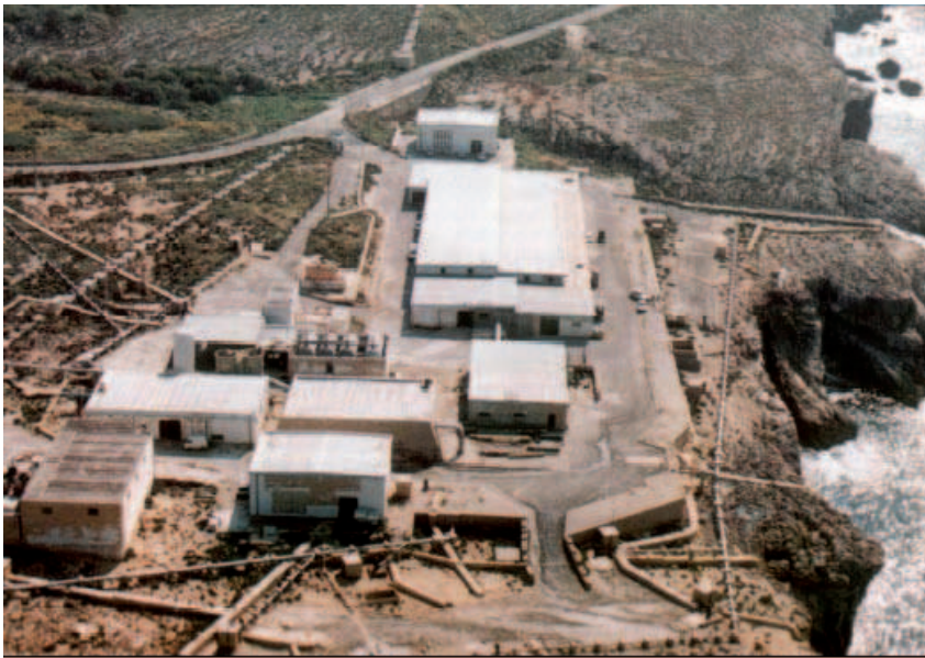
Figure 8. Reverse Osmosis Desalination Plant at Ghar Lapsi.
