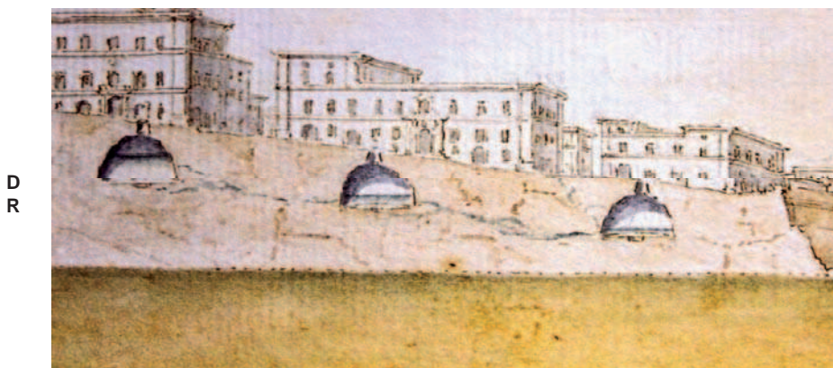
Figure 4. Detail from a watercolor depicting the construction of the new city of Valletta.
