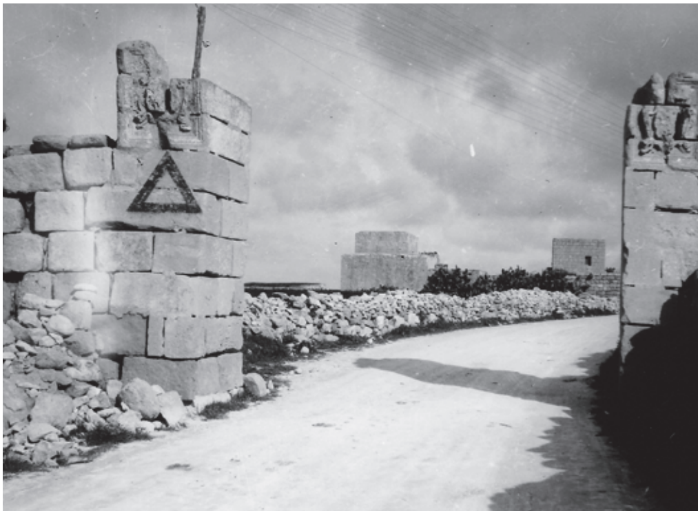
Fig. 12. Photograph dated 29 March 1933, taken from the north, of the pillars carrying armorial bearings that flanked the road through Ta’ Mrajġa at the point where it crossed the Falka Gap entrenchment.
